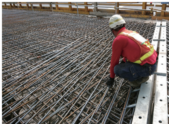
P423 橋面板鋼筋綁紮
