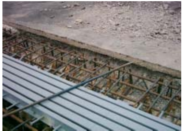
圖4.46 鬆動砂石清理後情形
