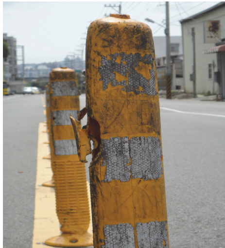
(b)受撞後破損
