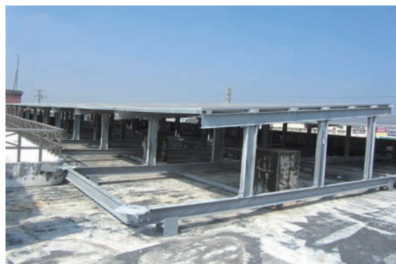
Setting up solar power panels on the roof
