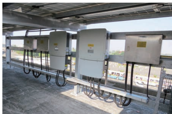
An inverter and a meter for solar powered equipment
