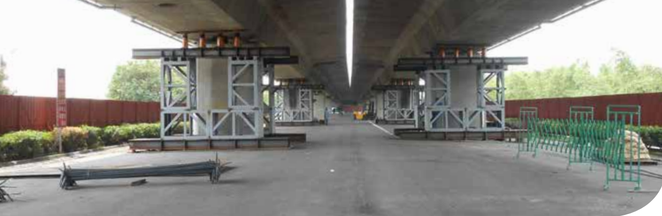
Temporarily shoring up the support frame for moving the main beam into position
