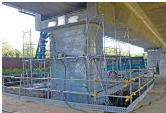
Bridge pier reinforcement construction
