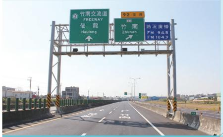
South bound 91K+900: The sign of name of interchange+ sign of Expressway exit+ sign of directions of the names of places+ markers of directions of the names of places
