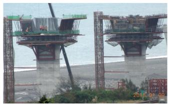
JinglunP9~P10 column top steel reinforcing bar binding and internal mold support installation
