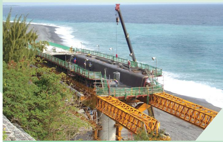
Duoliang U2-2 (P6~P7) Box beam and steel reinforcing bar binding
