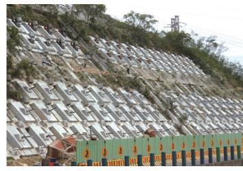
Provincial Highway 62 7K+140~7K+760 dip slope reinforcement
