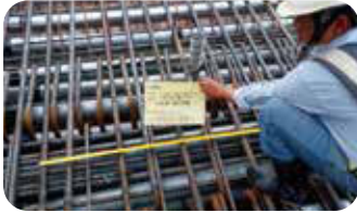
10.鋼筋及套管查驗
