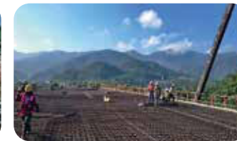
5. 頂板鋼筋綁紮
