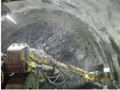
● 103.08.03 T703輪鏡面岩性完整
