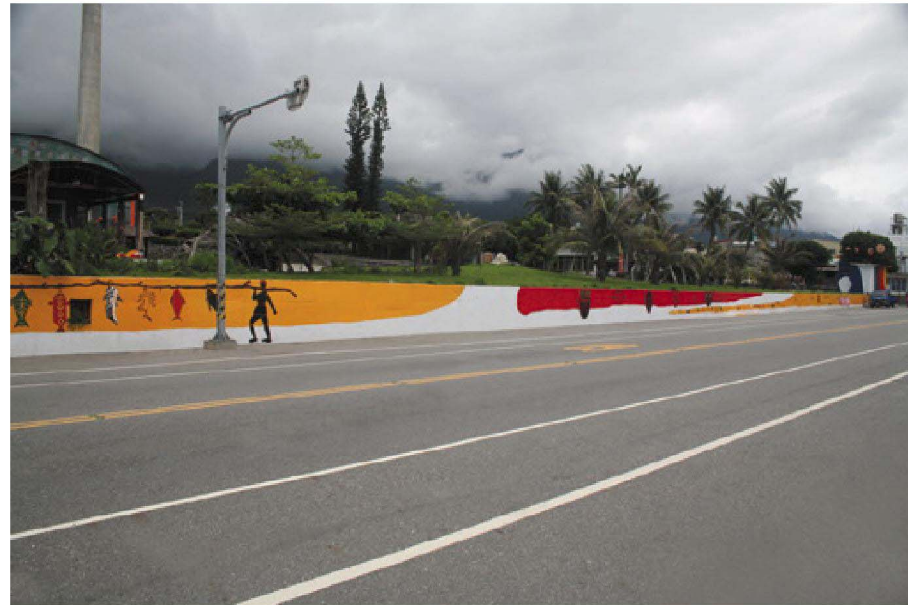
119 臺11線147K Taiwan Provincial Highway No.11 147K
