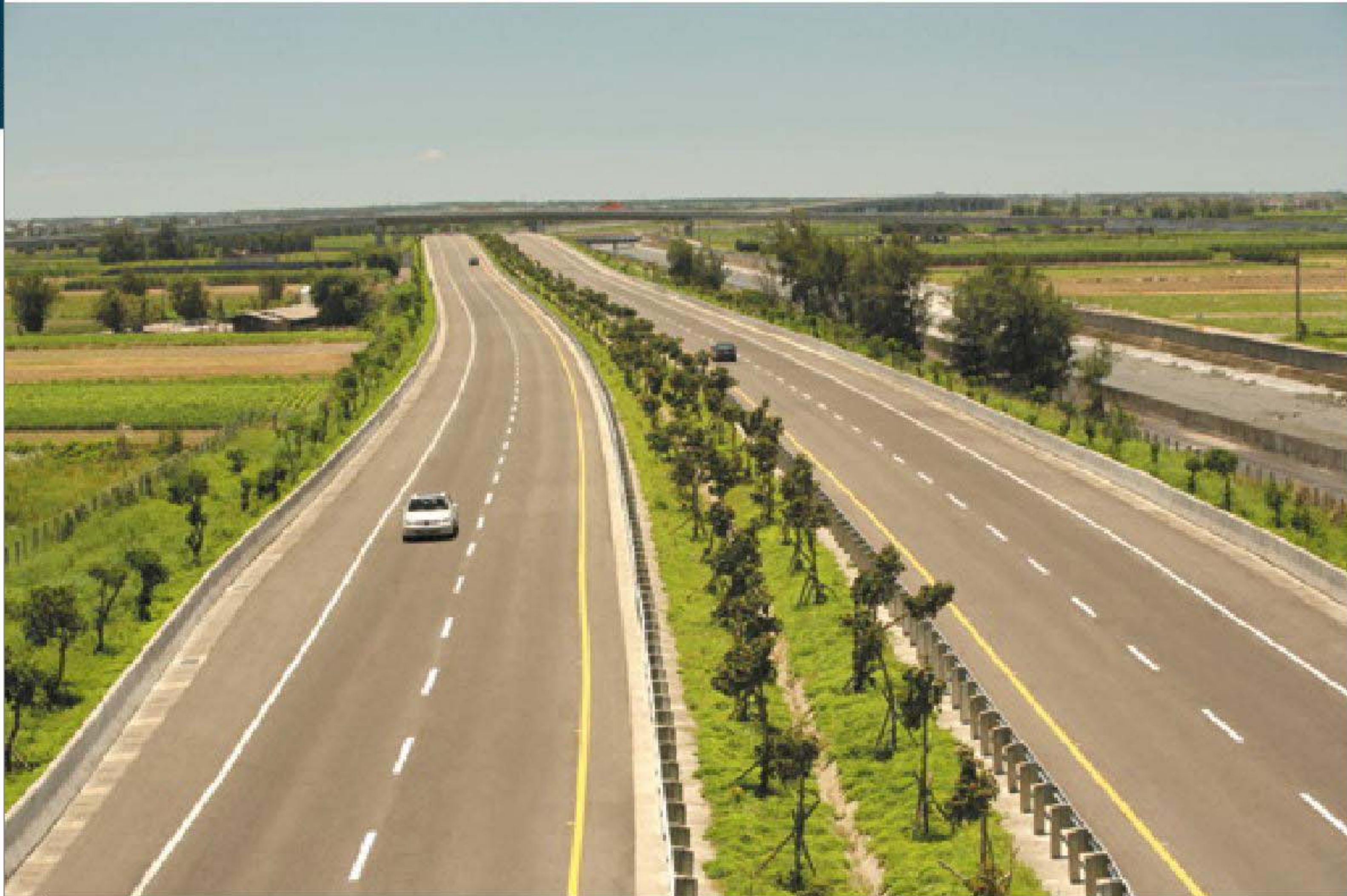
42 臺78線4.1K Taiwan Provincial Highway No. 78 4.1K
