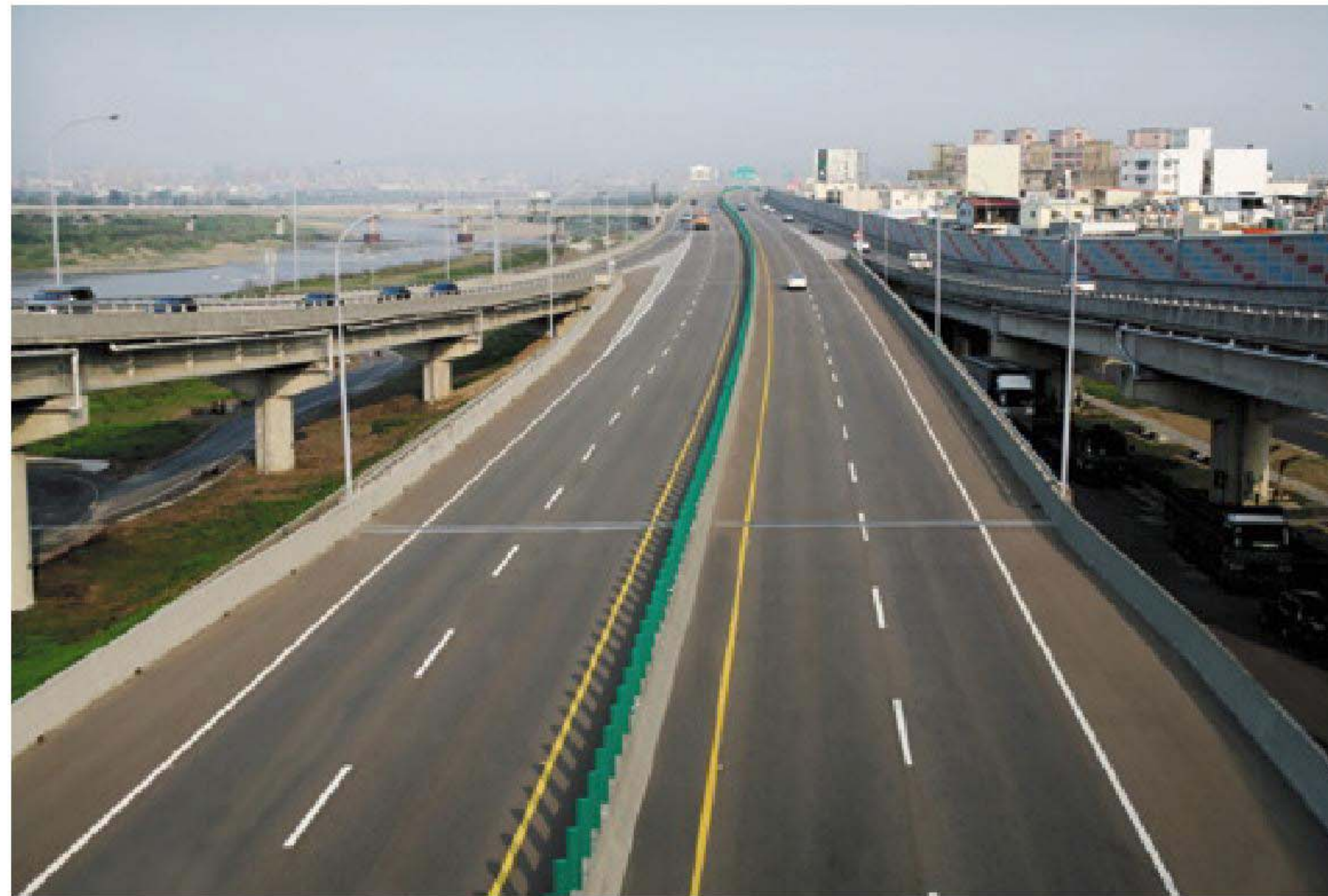
臺68線5K Taiwan Provincial Highway No. 68 5K
