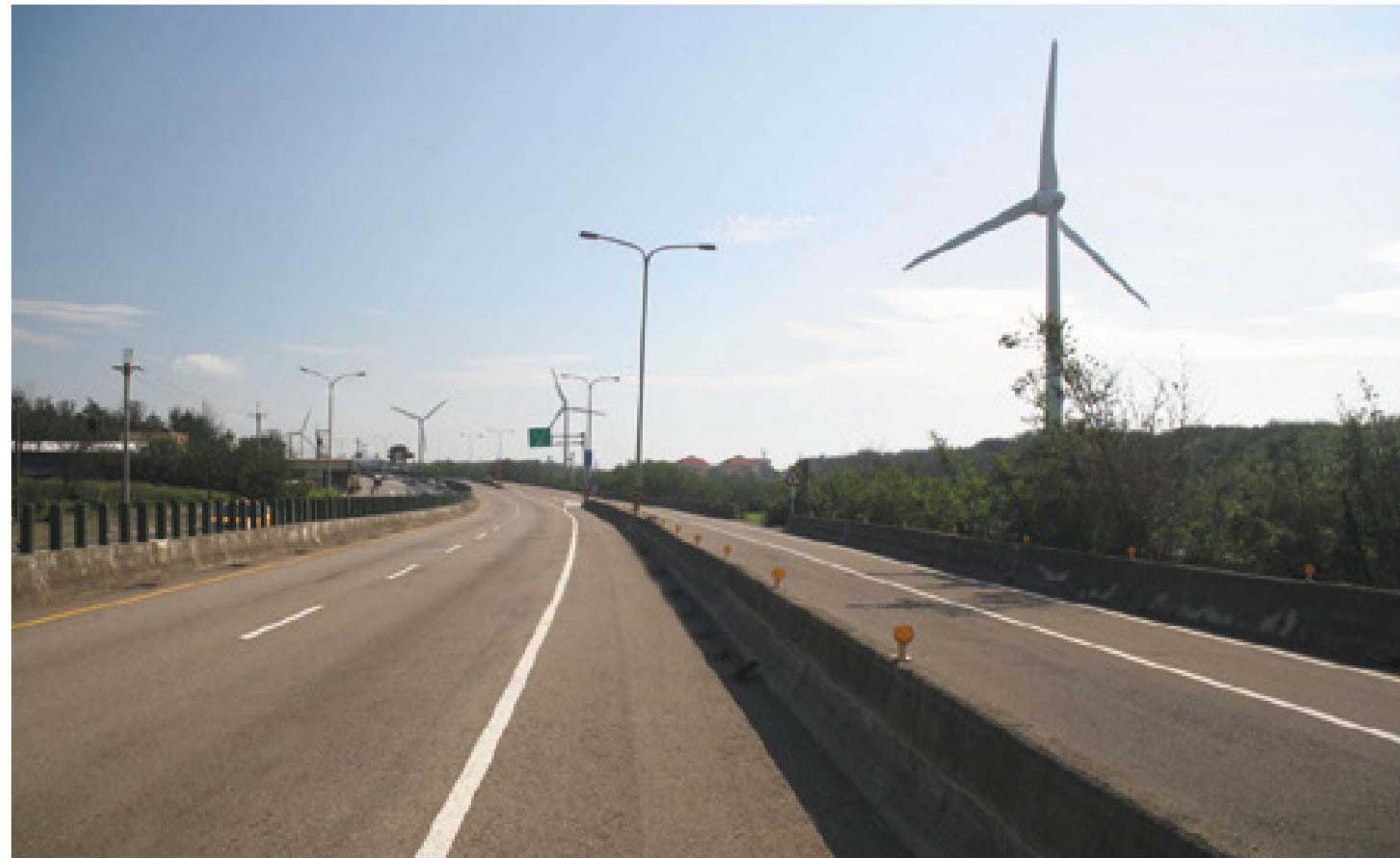
68 臺61線45K Taiwan Provincial Highway No.61 45K
