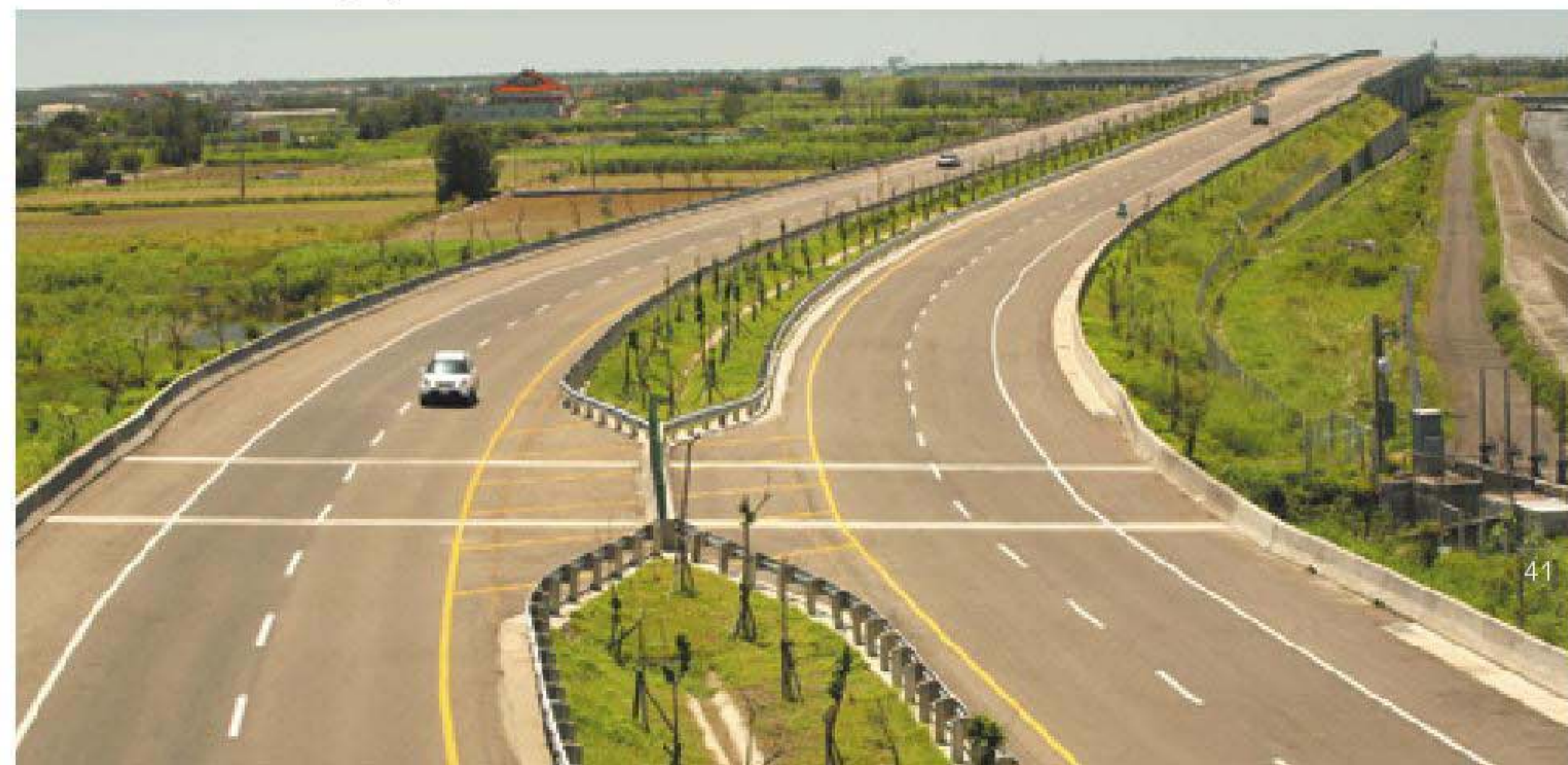
臺78線3K Taiwan Provincial Highway No.78 3K
