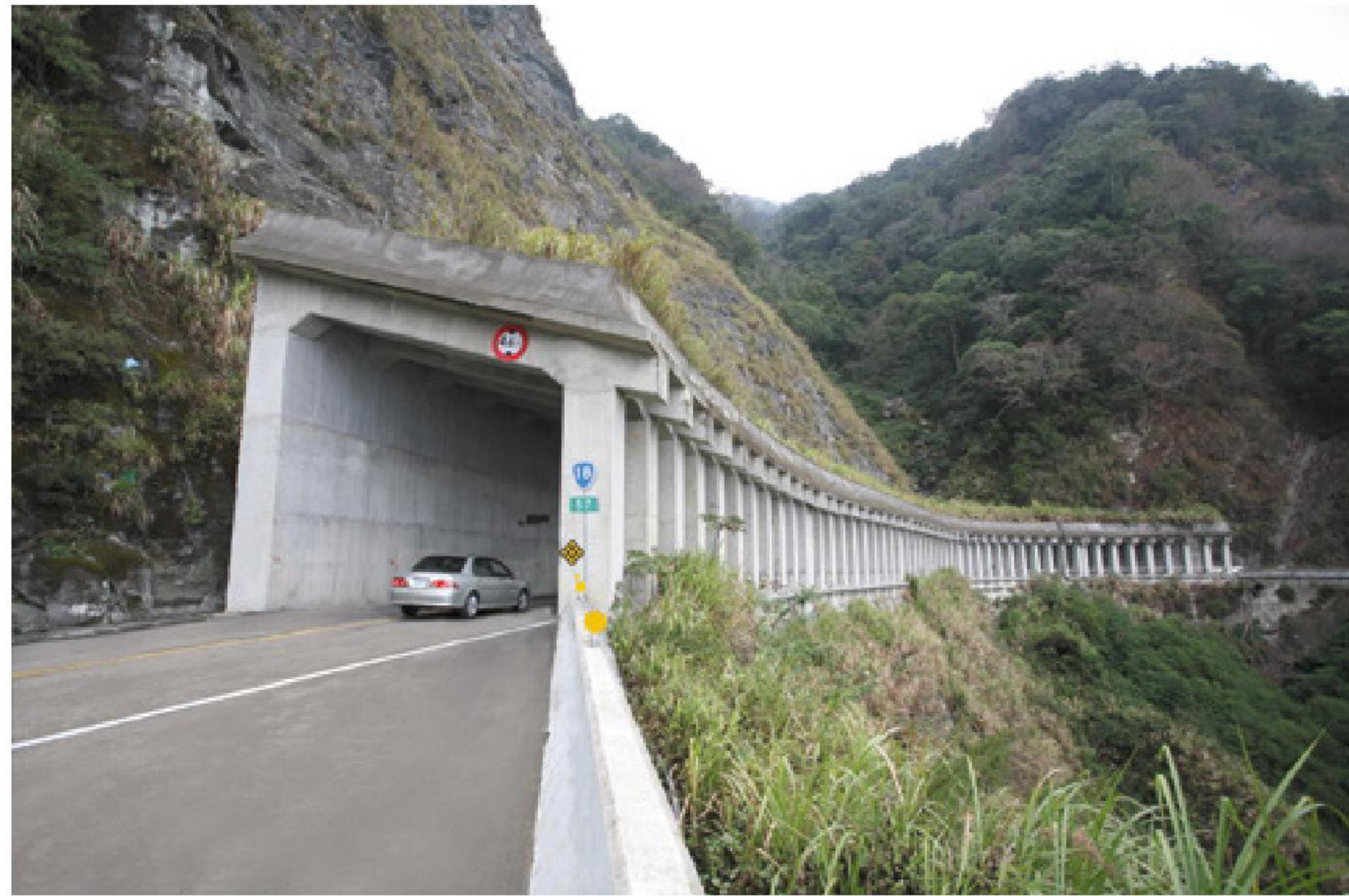
臺18線57K明隧道 The Open Tunnel on Taiwan Provincial Highway No.18 at 57K
