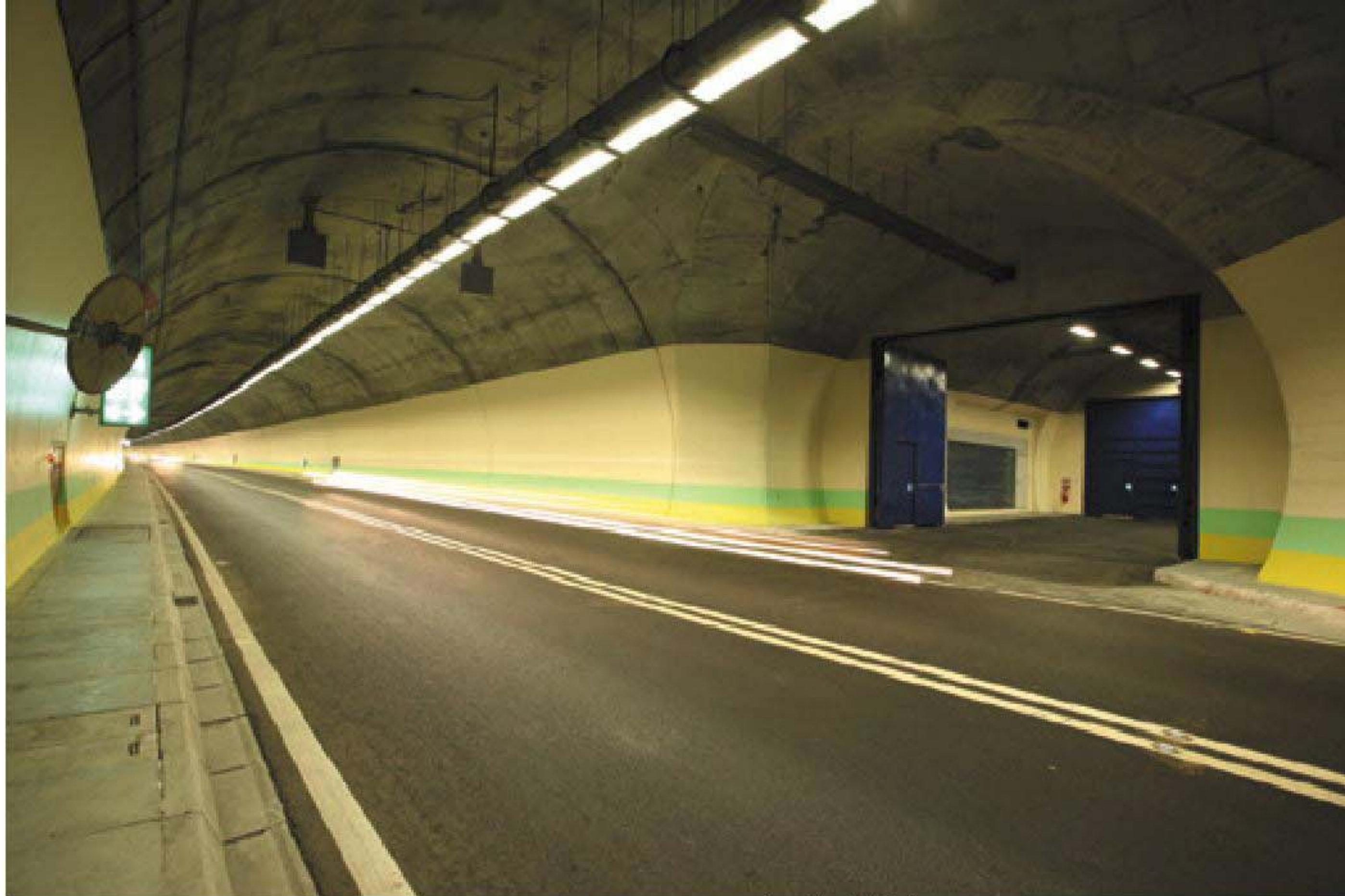
臺76線八卦山隧道 Taiwan Provincial Highway No.76 Baguashan Tunnel
