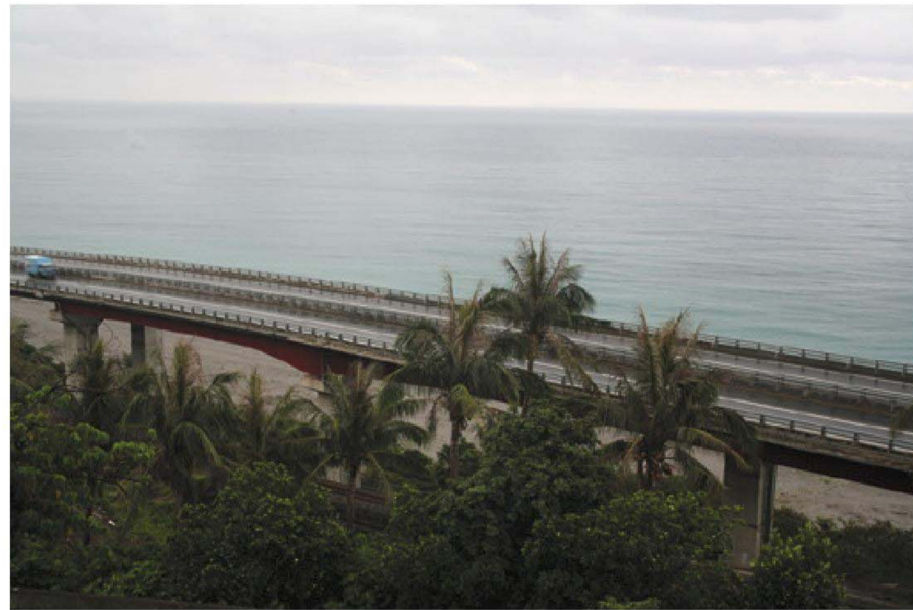
臺9線396K Taiwan Provincial Highway No.9 396K
