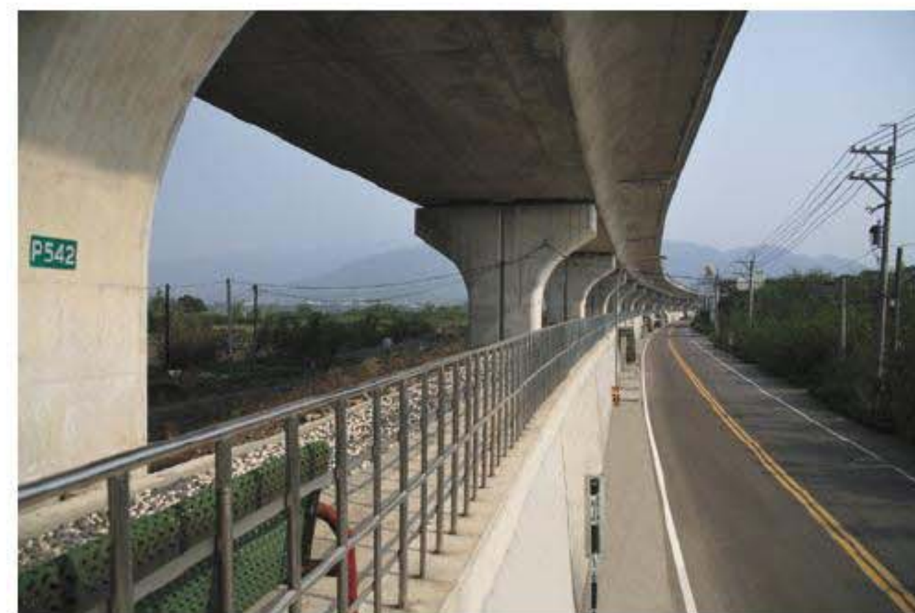
臺68線22.5K Taiwan Provincial Highway No.68 22.5K
