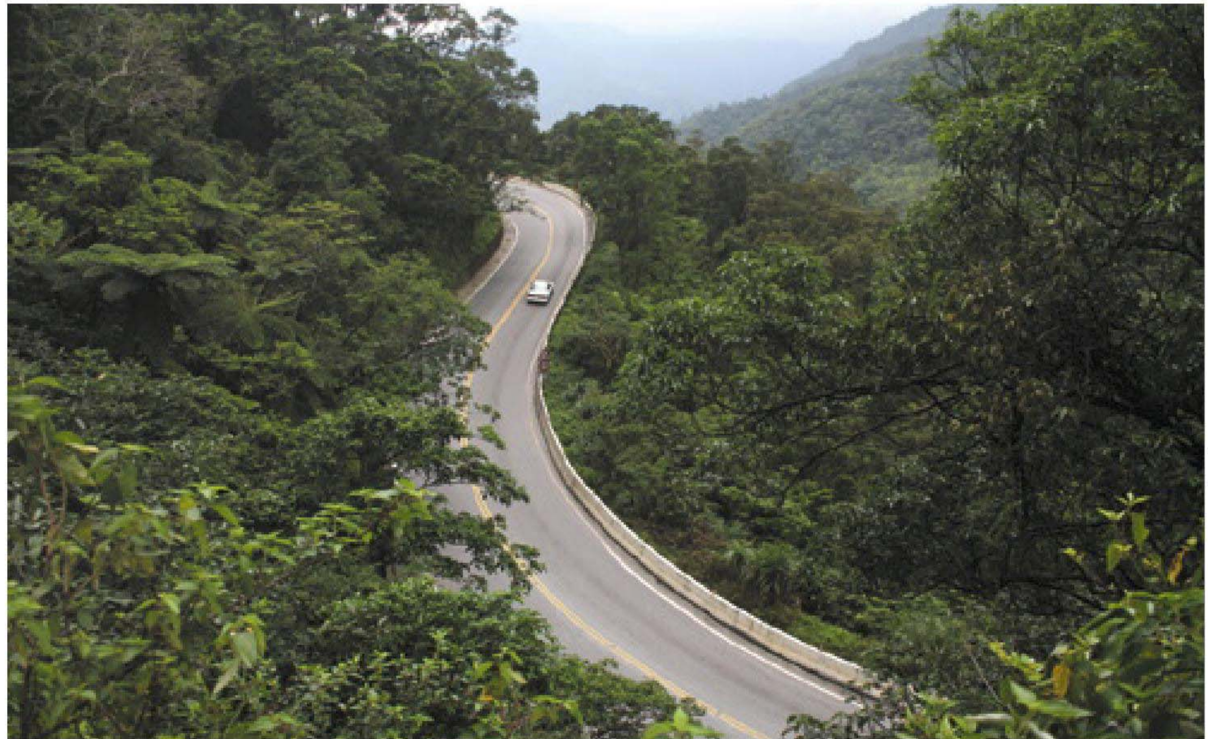
臺9線蘇花公路127.5K The Suhsua Highway of Taiwan Provincial Highway No.9 127.5K
