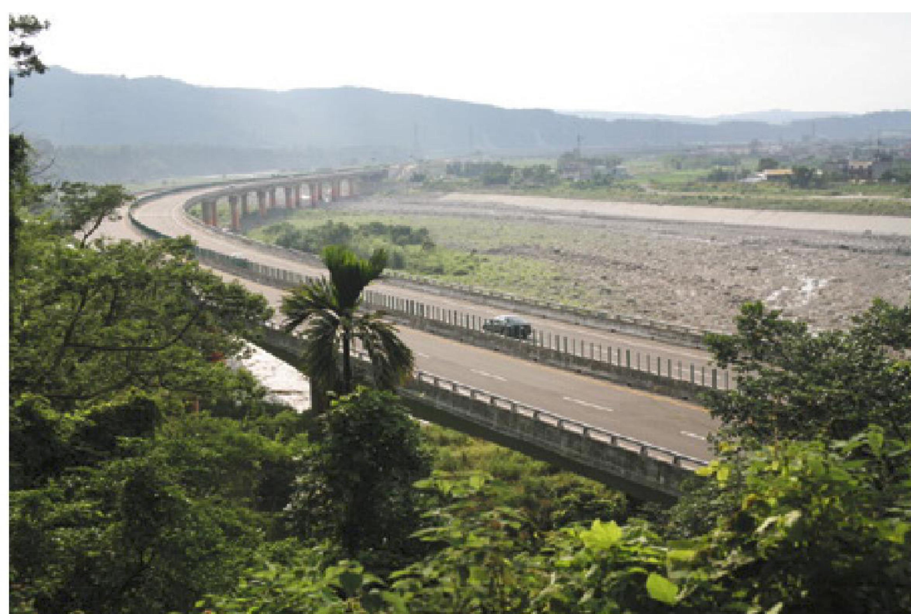
臺72線25K Taiwan Provincial Highway No.72 25K
