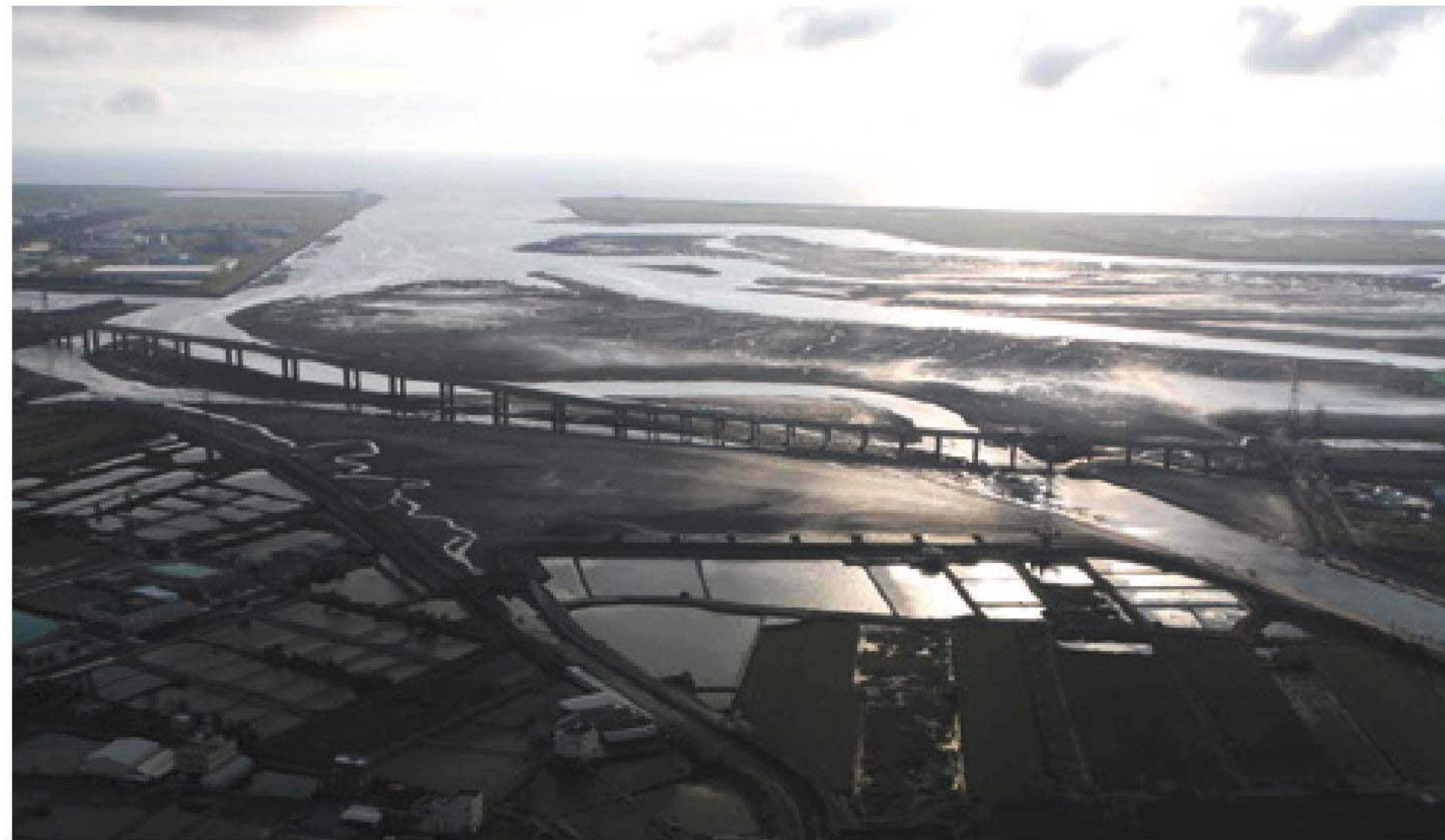
臺61線崙尾灣橋 Kuenwei Bay Bridge on Taiwan Provincial Highway No.61
