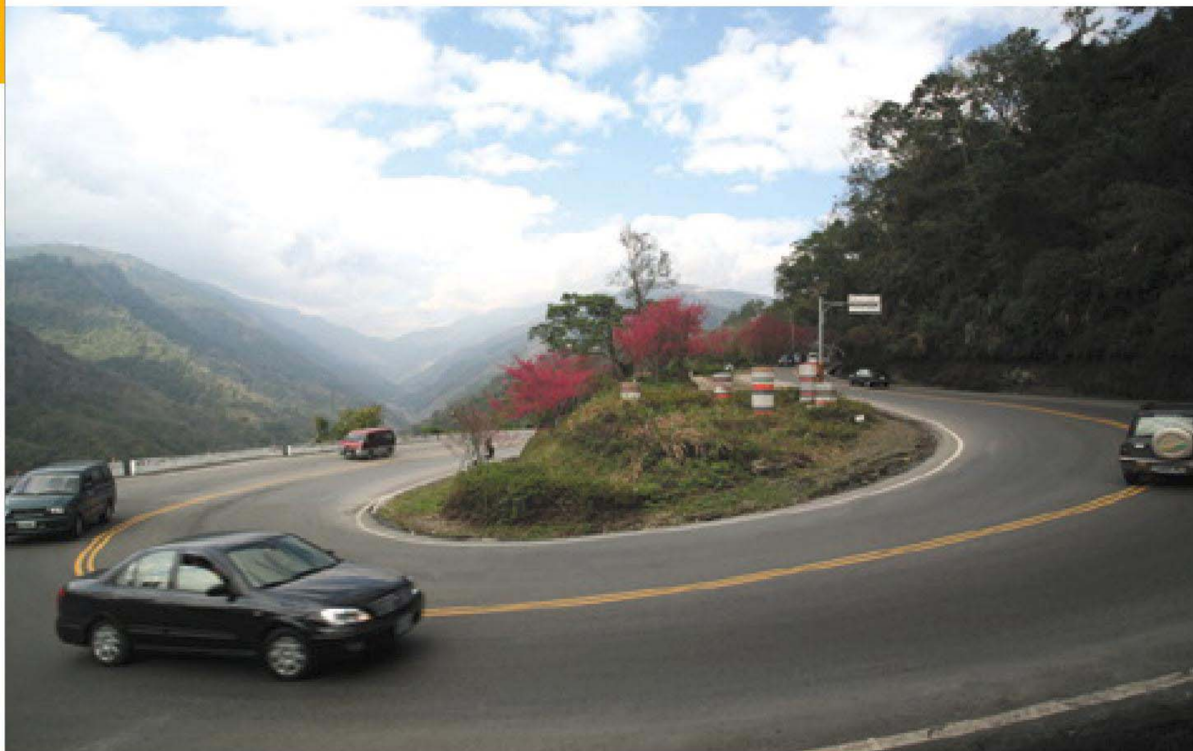
150 臺14線埔霧公路77.5K The Puwu Highway of Taiwan Provincial Highway No.14 77.5K
