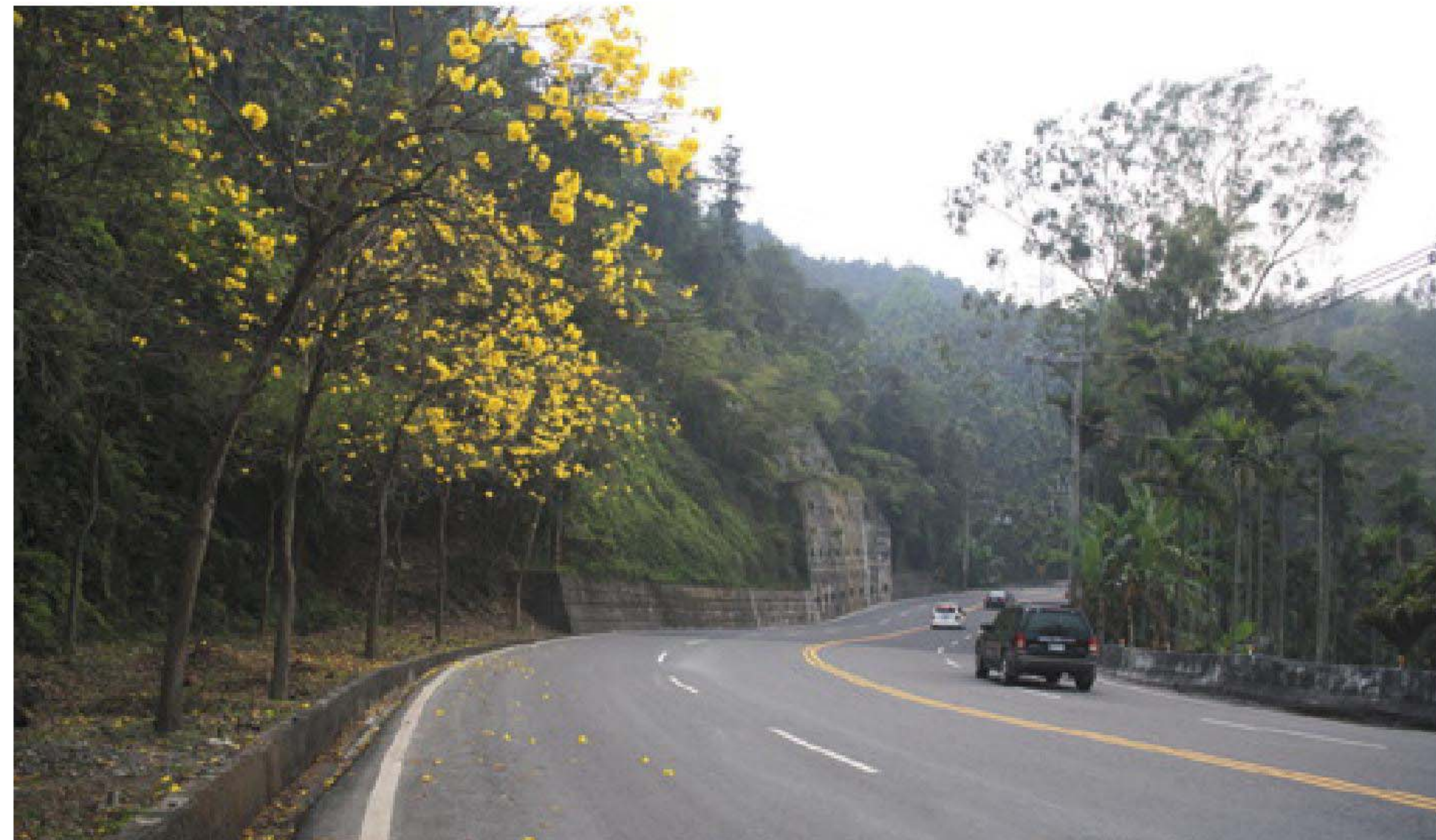
臺21線63K Taiwan Provincial Highway No.21 63K
