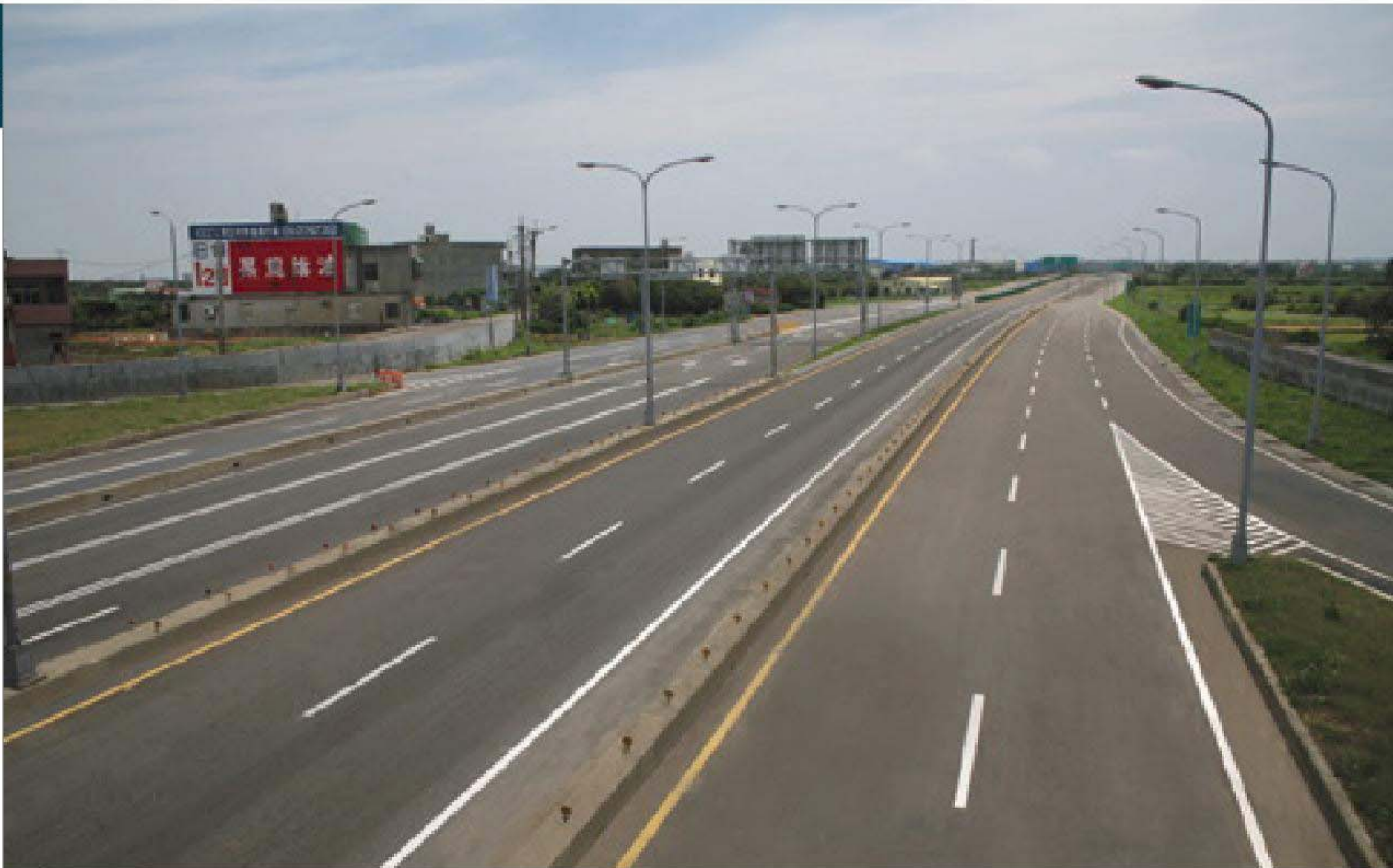
12 臺66線1.5K Taiwan Provincial Highway No.66 1.5K
