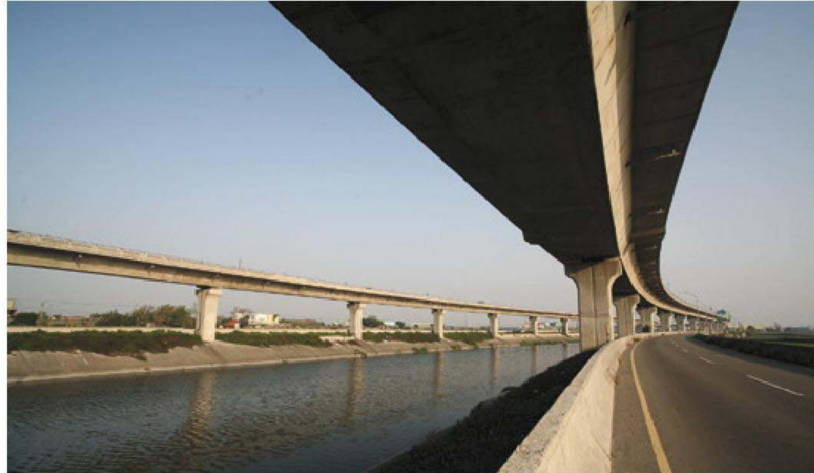
臺76線16K Taiwan Provincial Highway No. 76 16K
