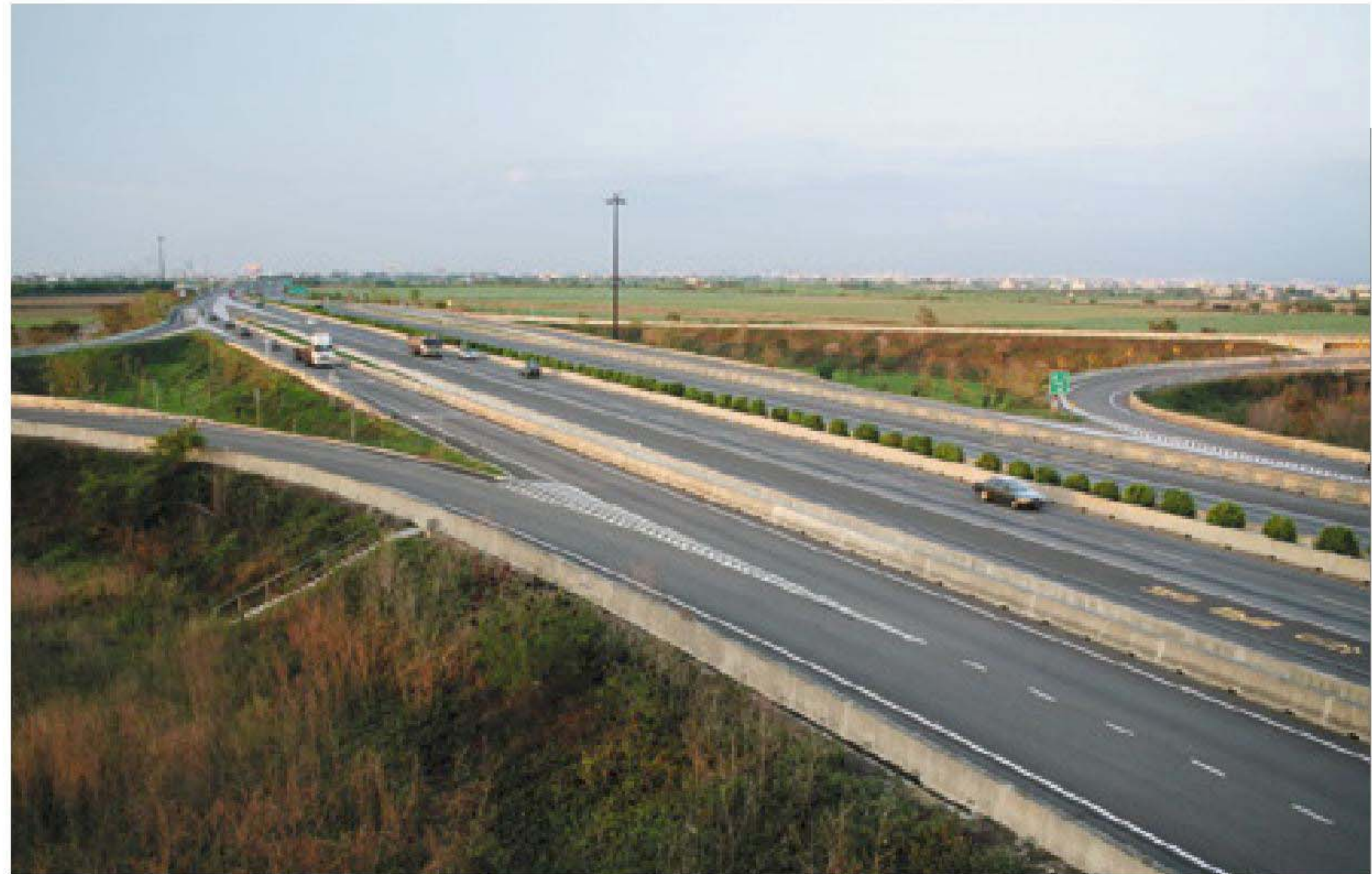
臺82線22K Taiwan Provincial Highway No.82 22K
