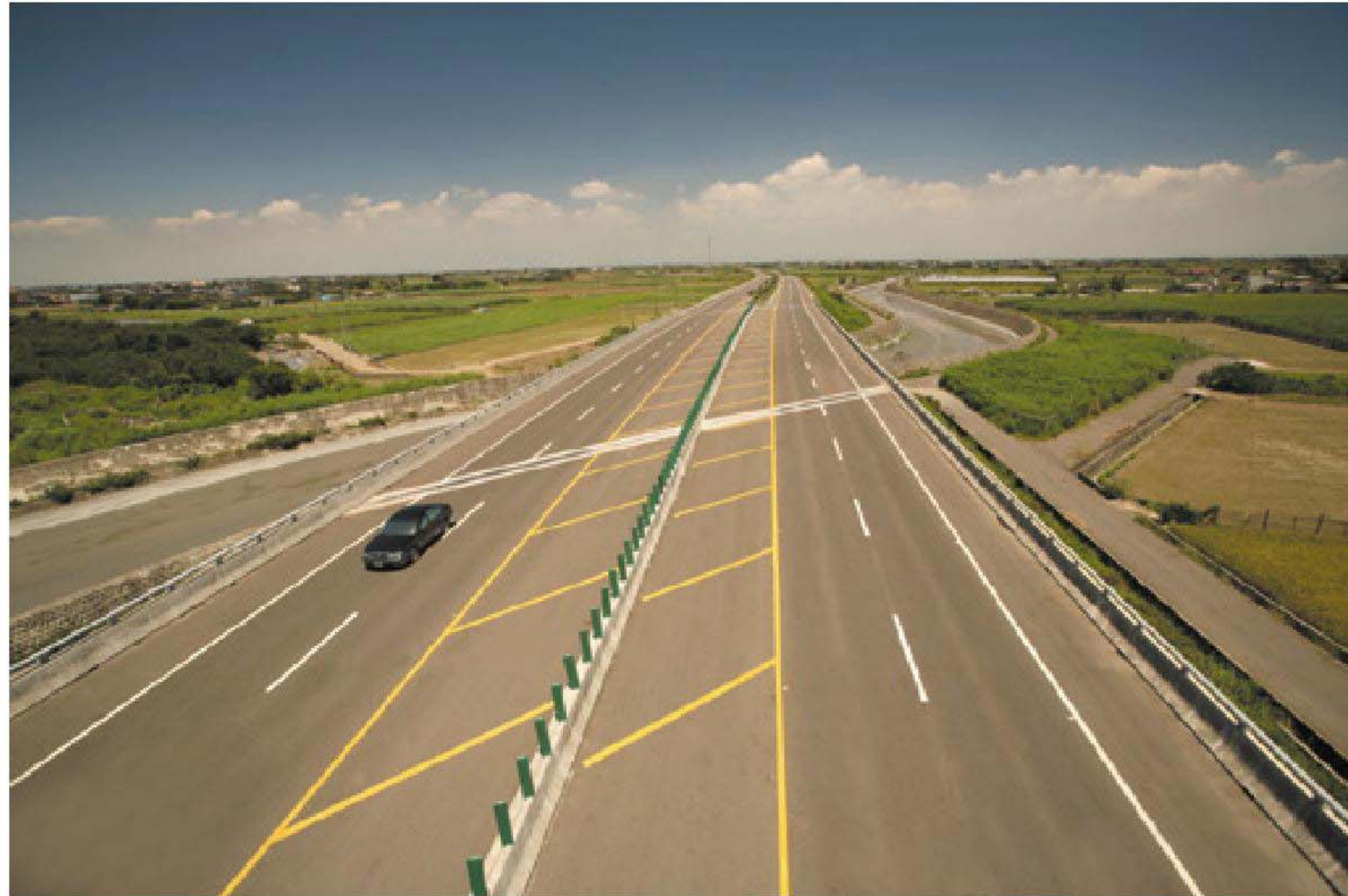
臺78線4.7K Taiwan Provincial Highway No. 78 4.7K
