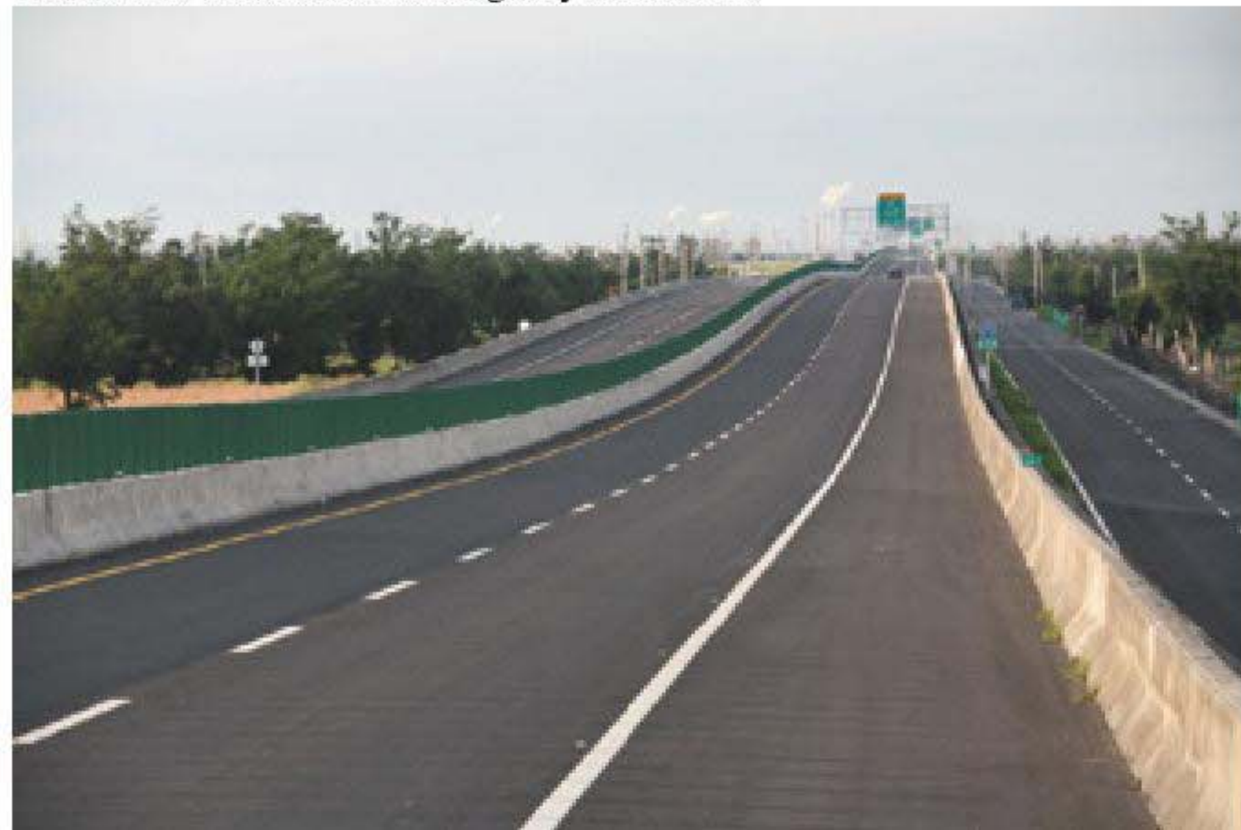
臺61線235K Taiwan Provincial Highway No.61 235K
