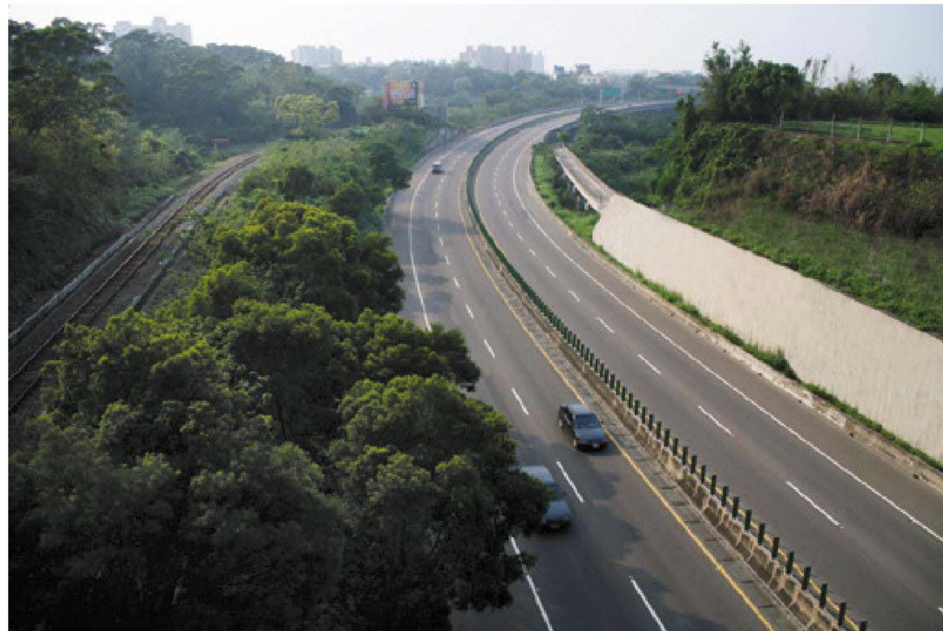
臺68線17K Taiwan Provincial Highway No.68 17K
