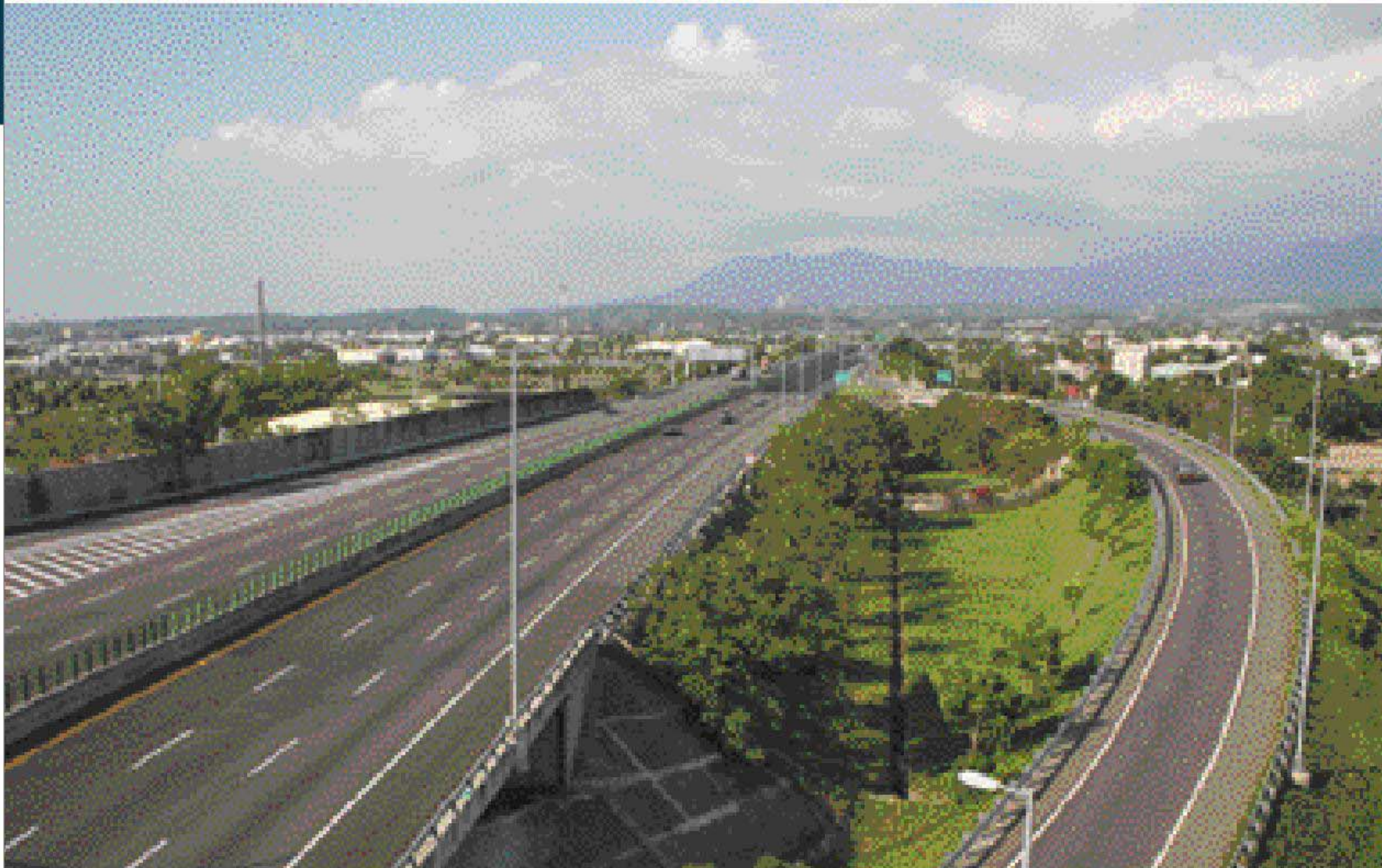
48 水上系統交流道 (國道3/臺82) Shueishang Interchange System (National Freeway No.3 / Taiwan Provincial Highway No.82)
