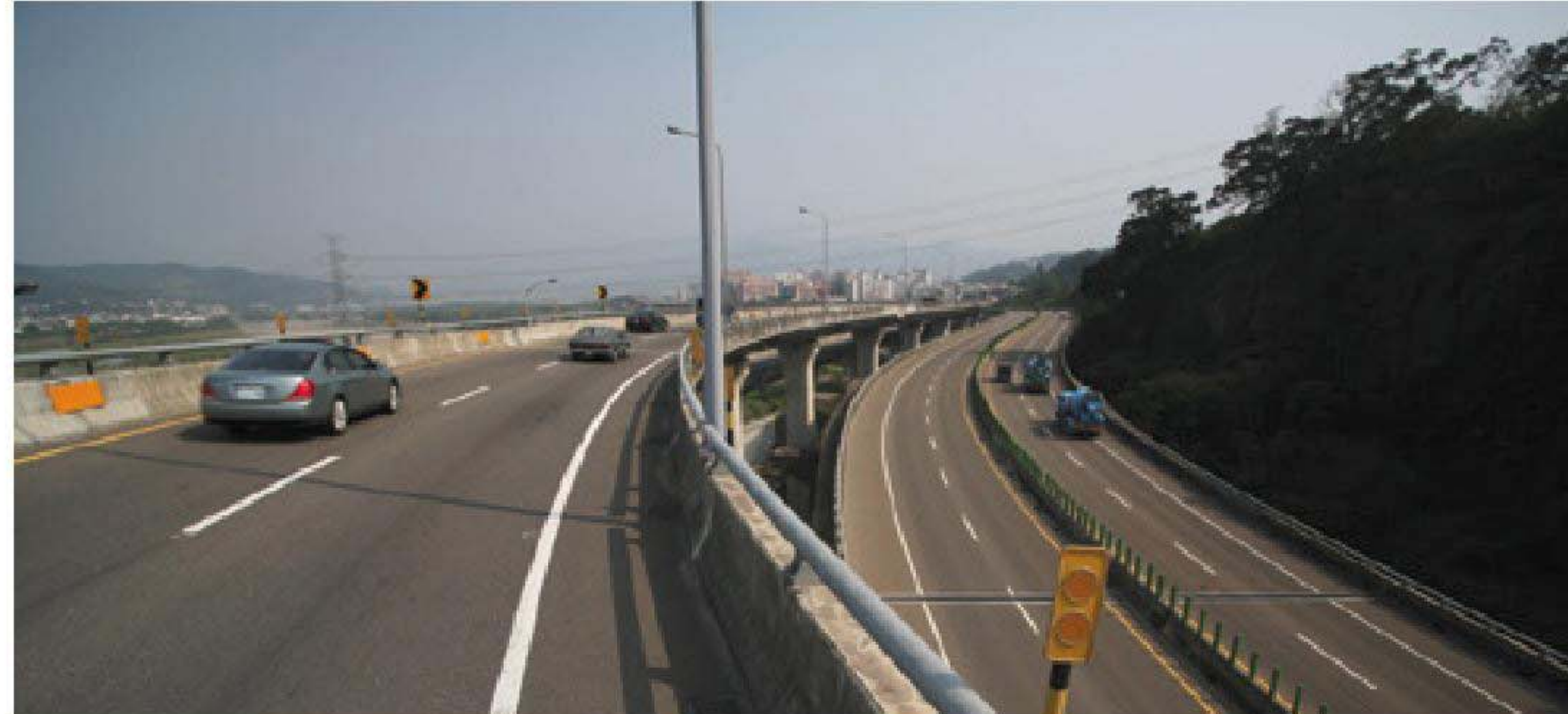
臺68線19K Taiwan Provincial Highway No.68 19K
