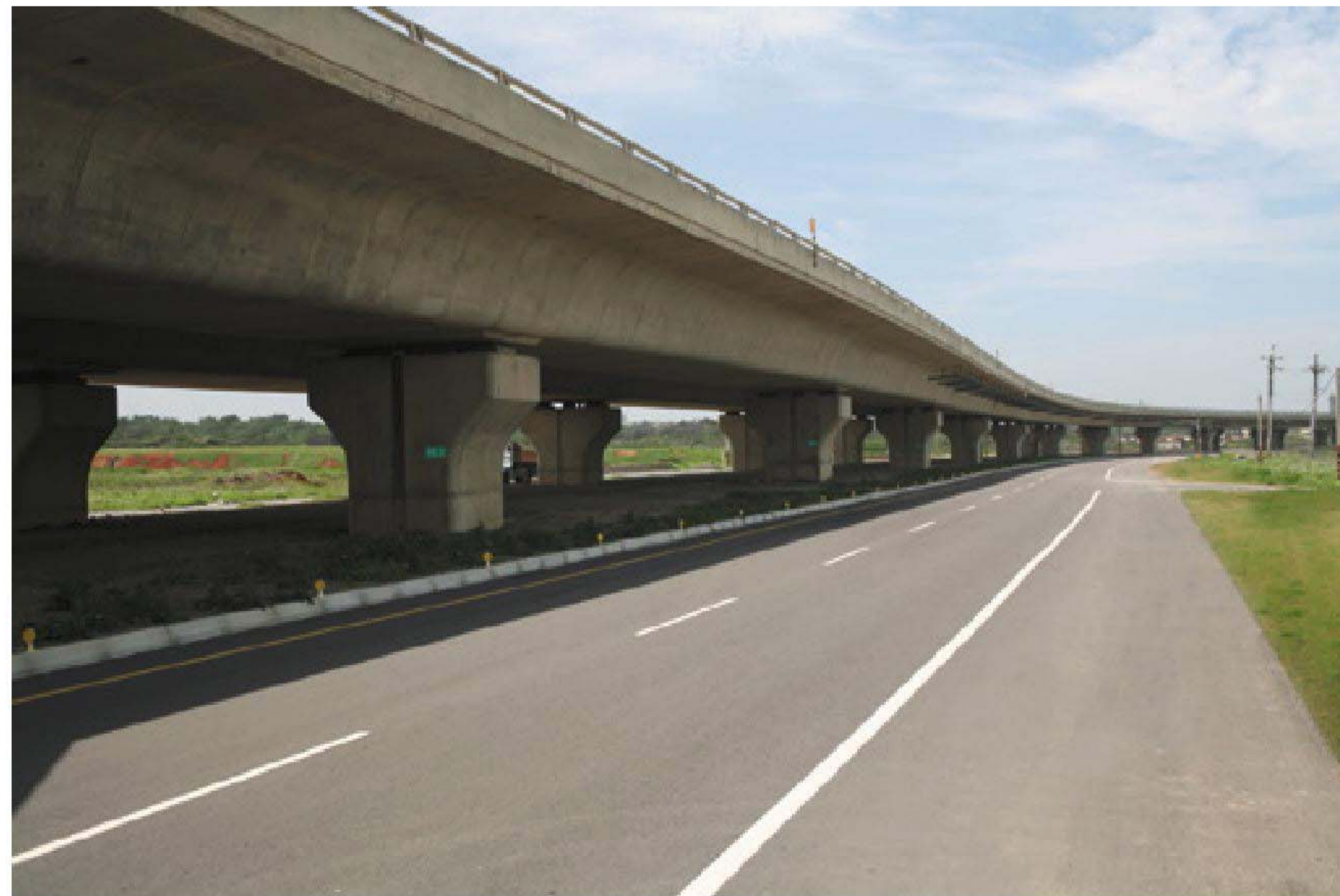
臺61線24K Taiwan Provincial Highway No.61 24K
