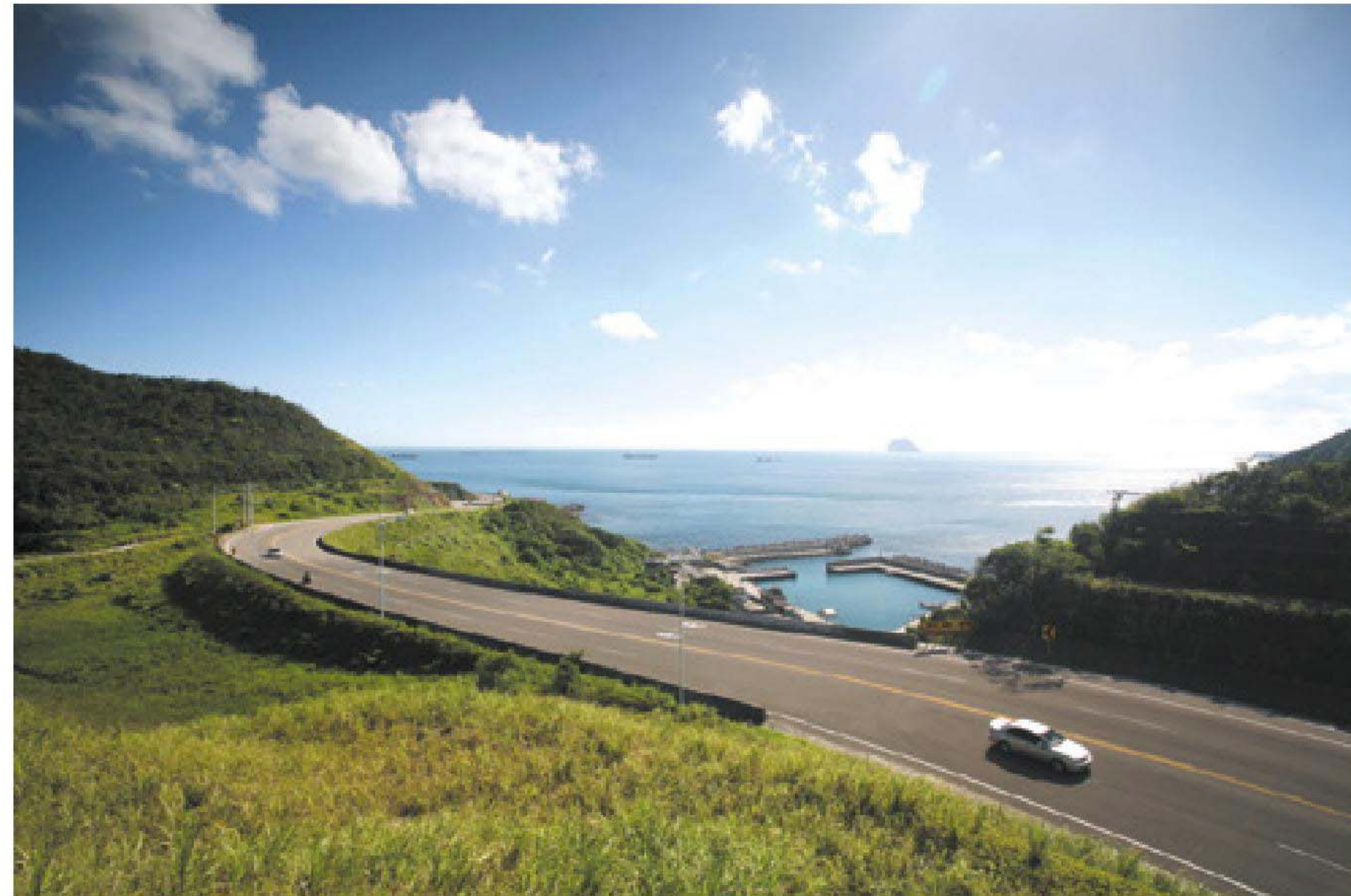
85 臺2線53K Taiwan Provincial Highway No.2 53K
