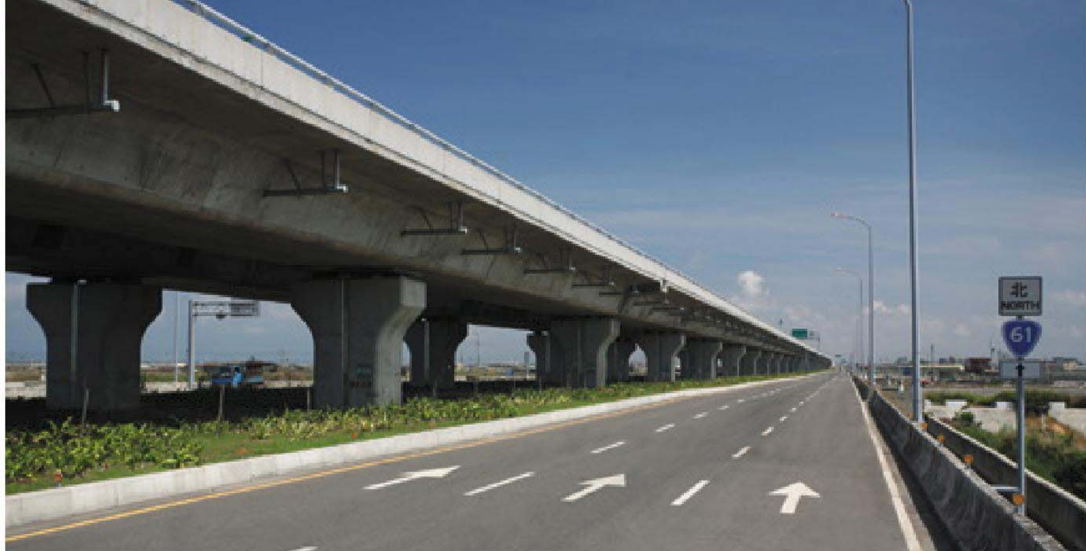
臺61線262K Taiwan Provincial Highway No.61 262K
