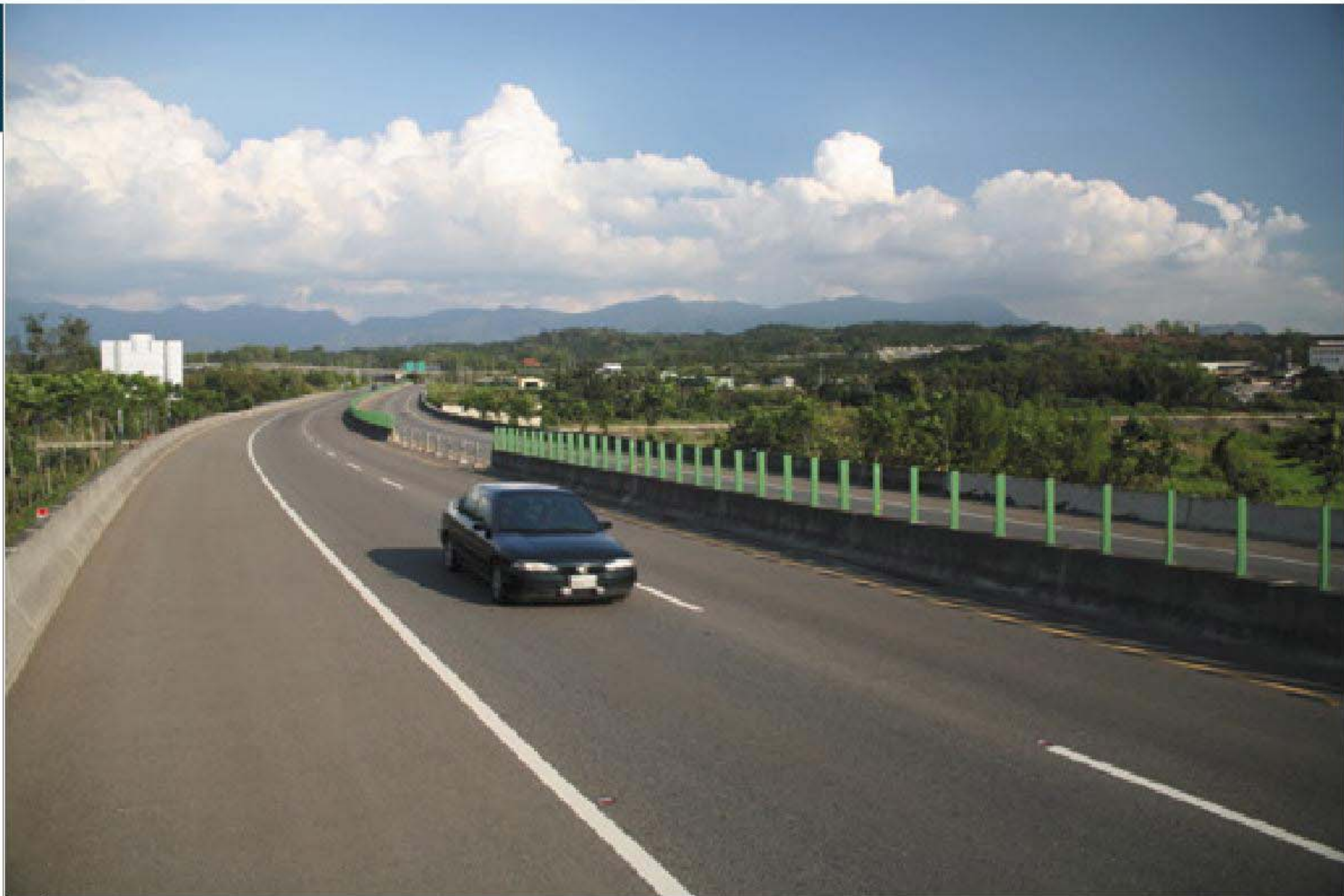
50 臺82線33.5K Taiwan Provincial Highway No.82 33.5K
