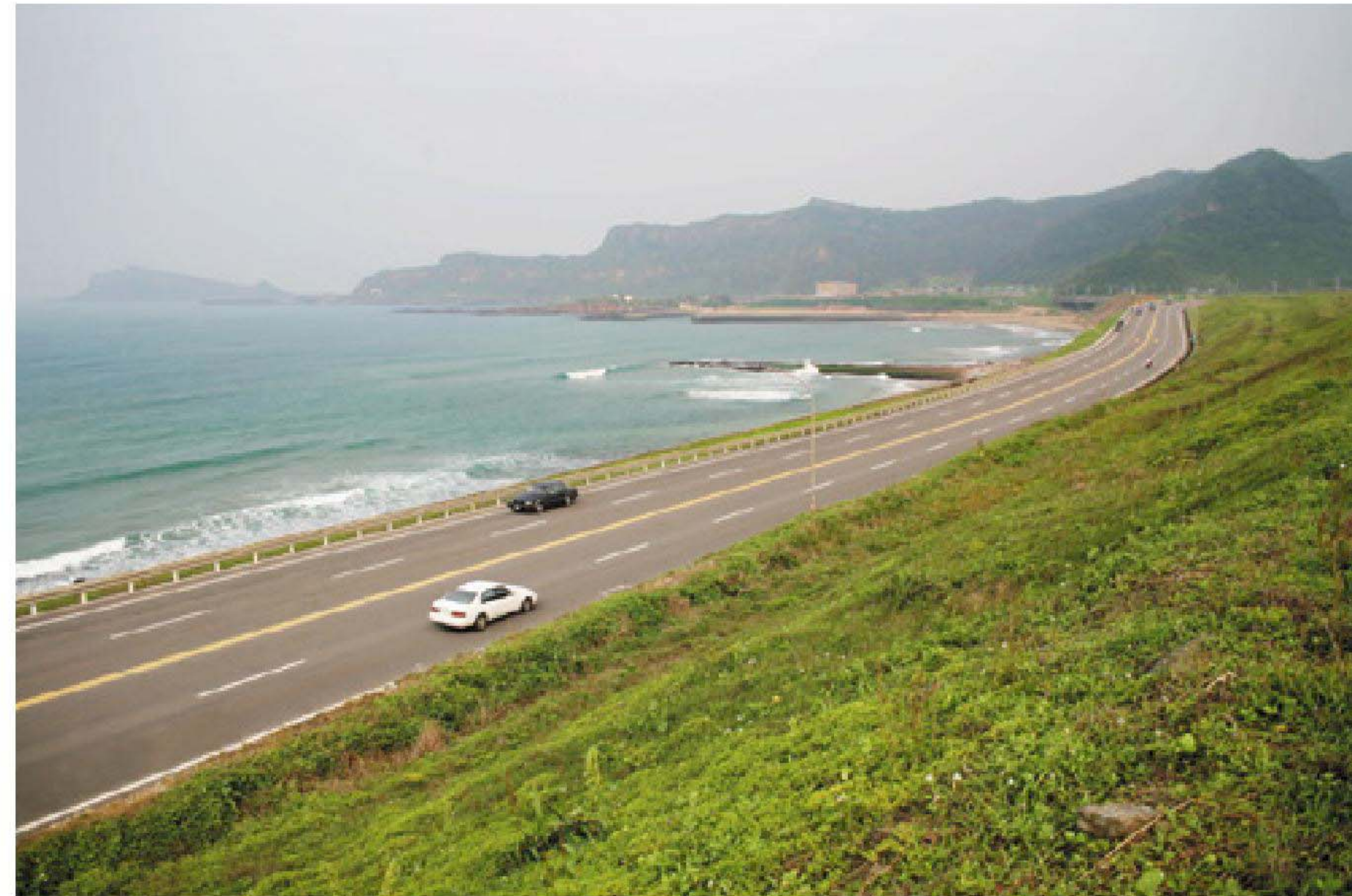
84 臺2線46K Taiwan Provincial Highway No.2 46K
