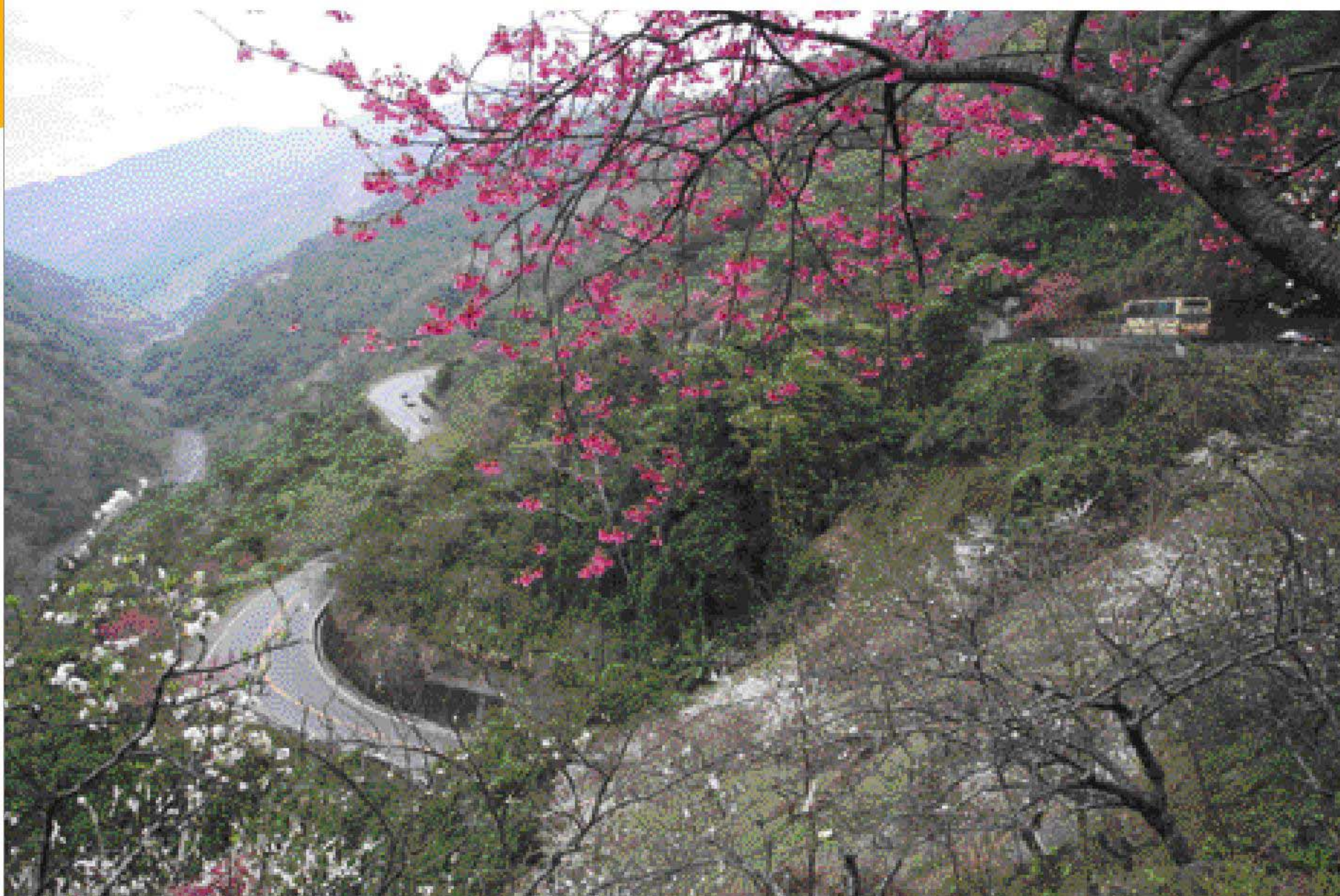
132 臺14線埔霧公路76.5K The Puwu Highway of Taiwan Provincial Highway No.14 76.5K
