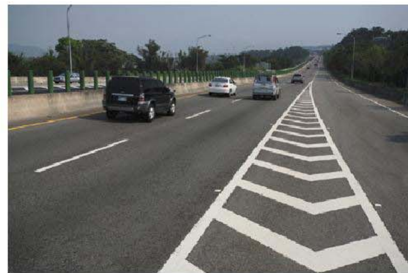
臺68線13.5K Taiwan Provincial Highway No.68 13.5K
