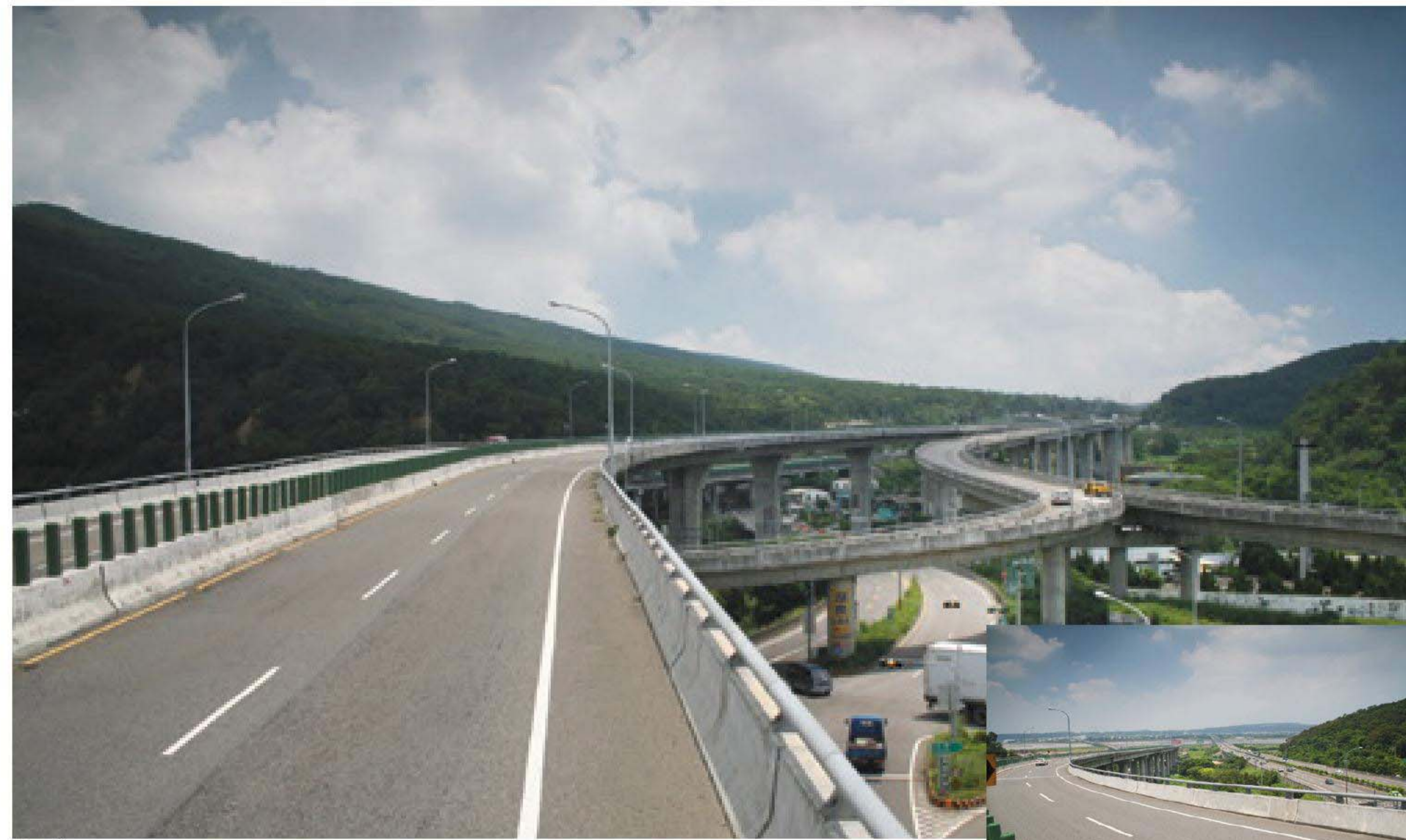
臺13線55.5K Taiwan Provincial Highway No.13 55.5K
