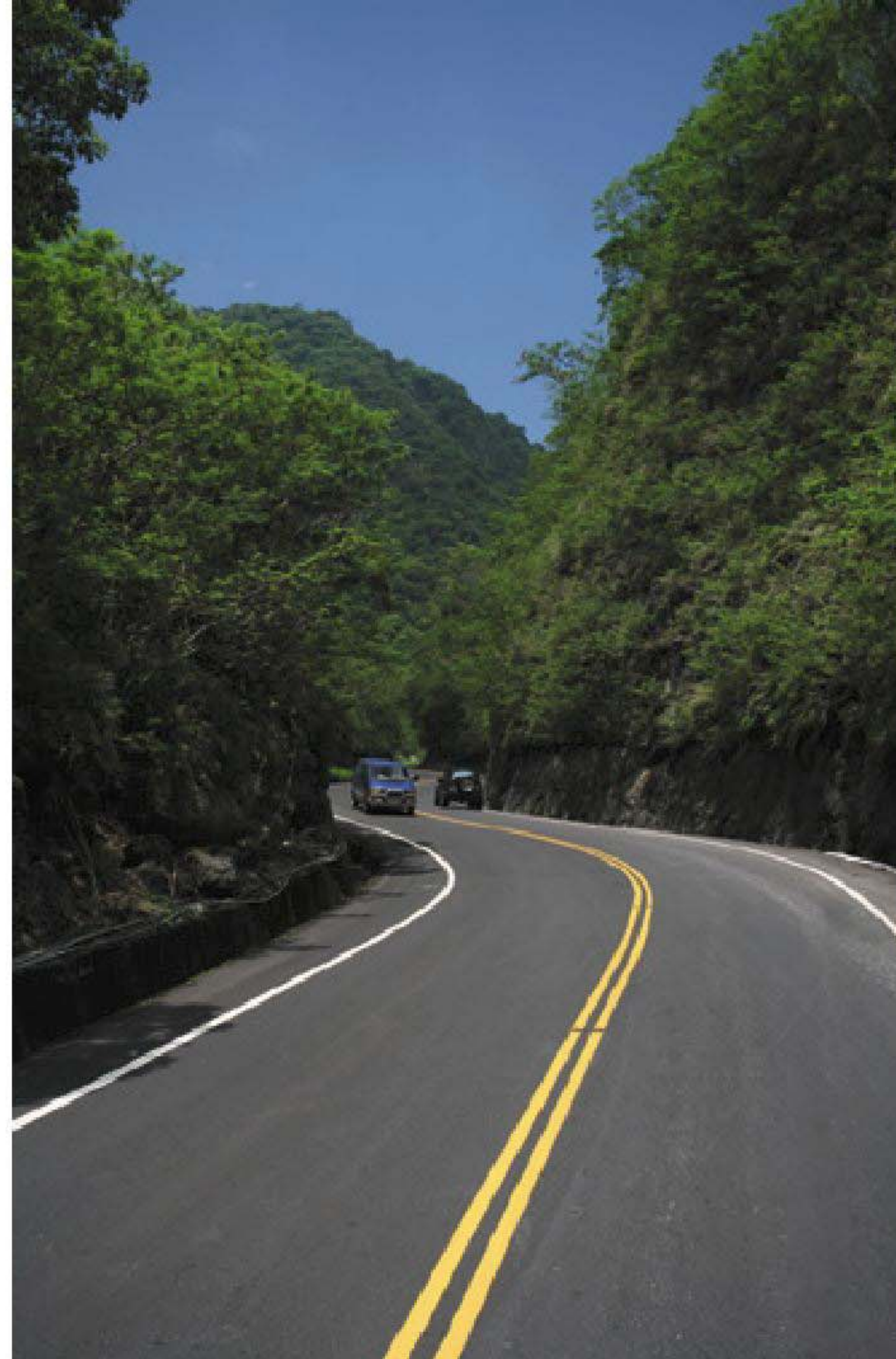
臺23線45K Taiwan Provincial Highway No.23 45K
