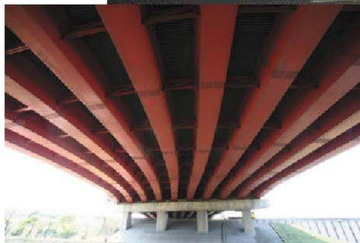
平鎮系統交流道鋼構箱型梁橋 Pingjhen Interchange System Steel Box Girder Bridge
