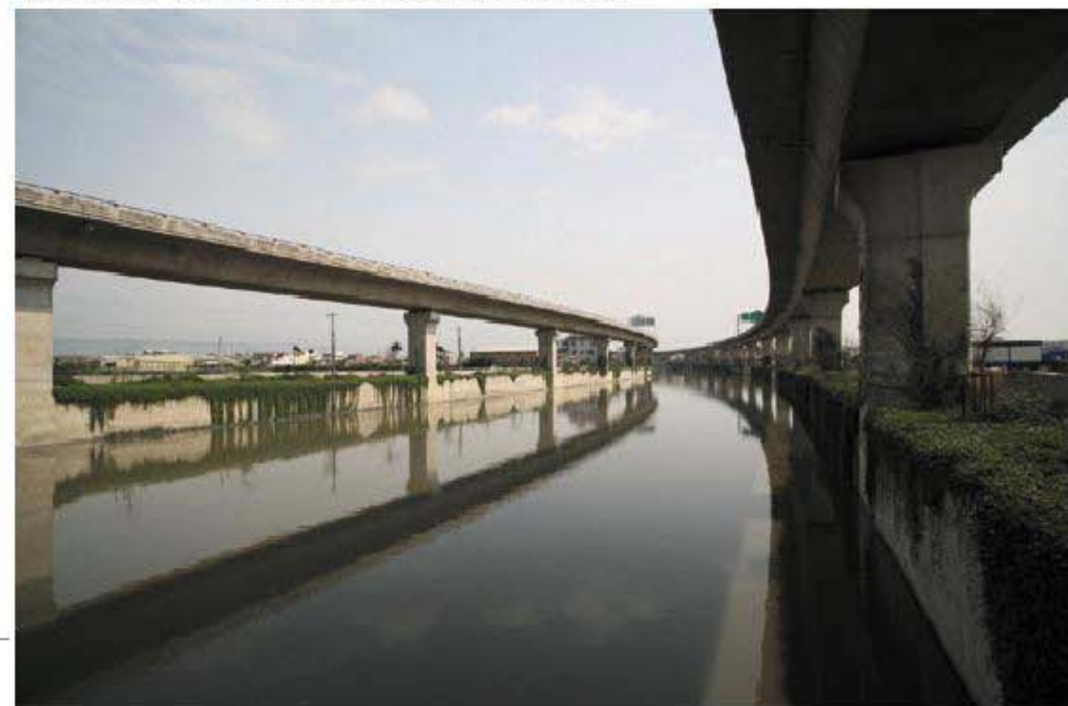
臺76線18K Taiwan Provincial Highway No.76 18K
