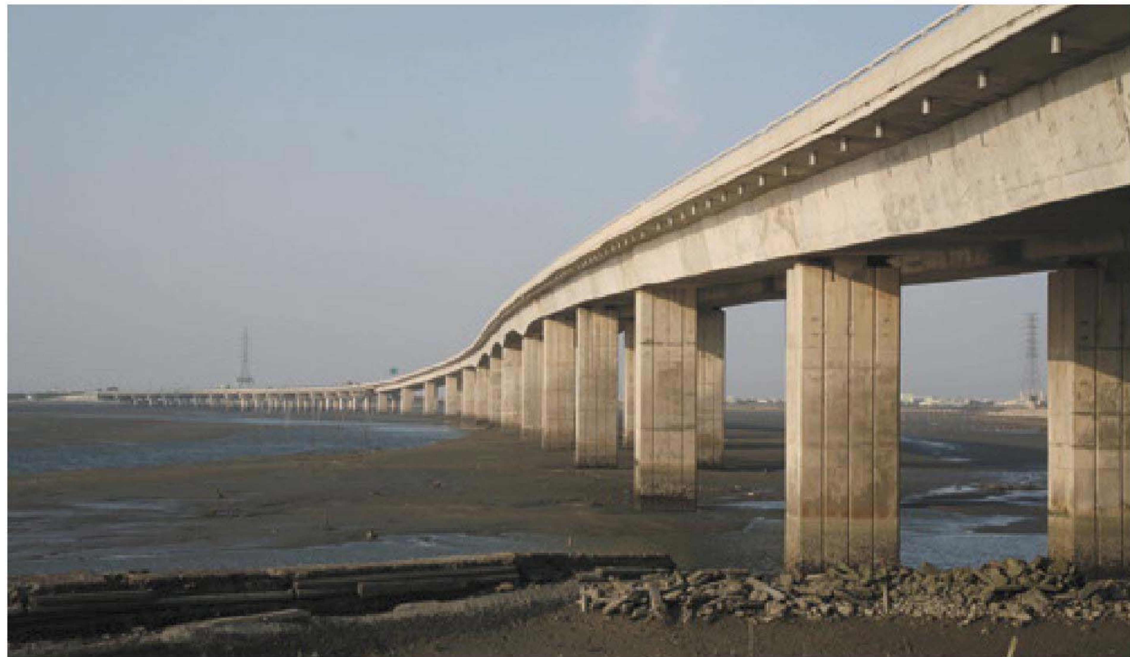
72 臺61線崙尾灣橋 Kuenwei Bay Bridge on Taiwan Provincial Highway No.61
