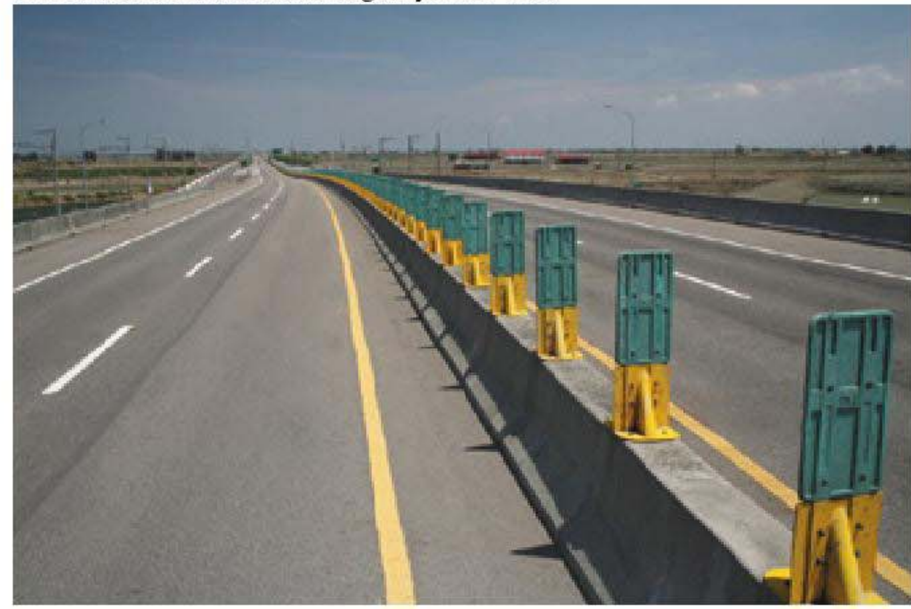
臺61線282K Taiwan Provincial Highway No.61 282K
