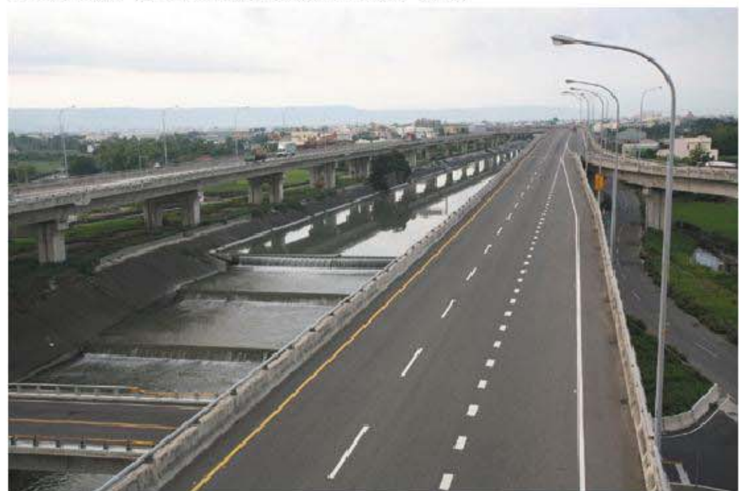
臺76線15.2K Taiwan Provincial Highway No.76 15.2K
