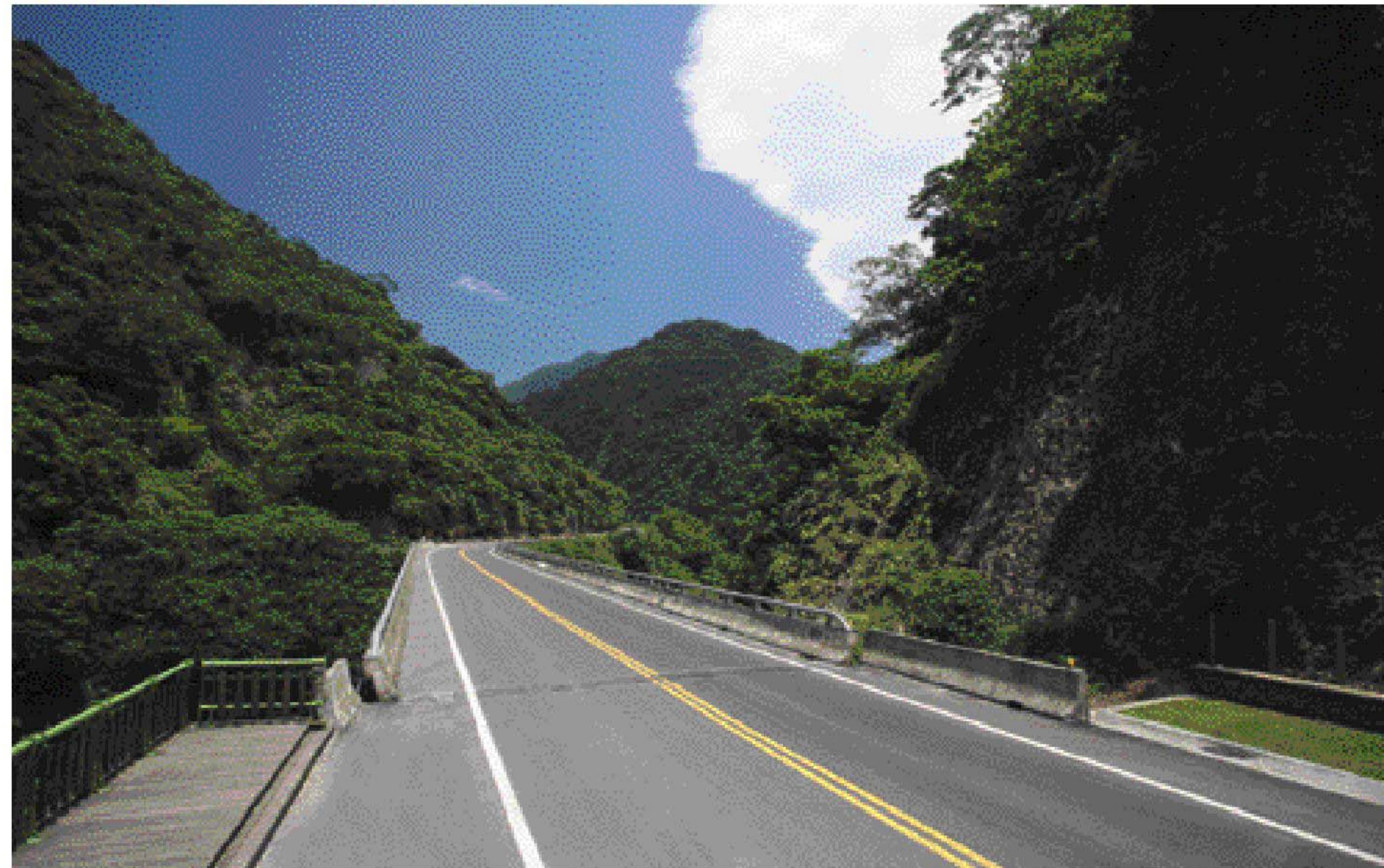
臺23線41K Taiwan Provincial Highway No.23 41K
