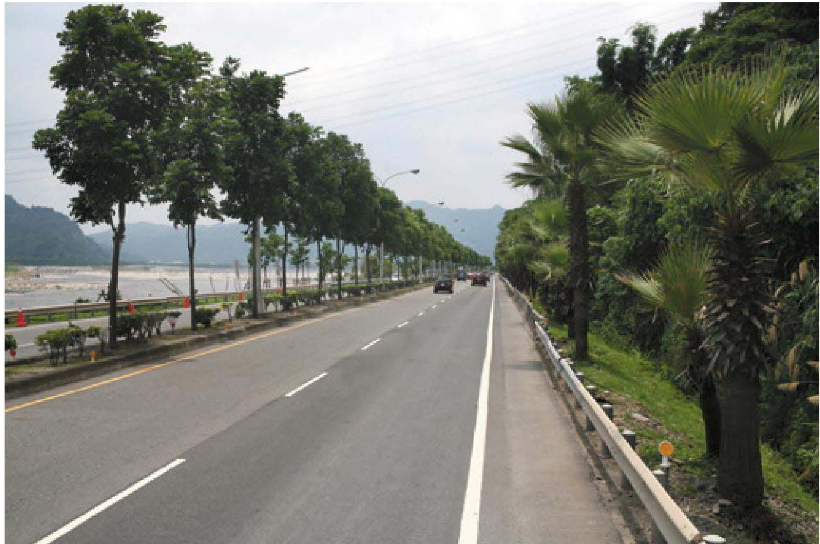
臺16線11.7K Taiwan Provincial Highway No.16 11.7K
