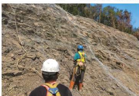
照0-04 格框鋪設菱型網及鋼筋
