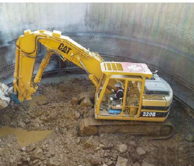
照0-80 豎井井口開挖
