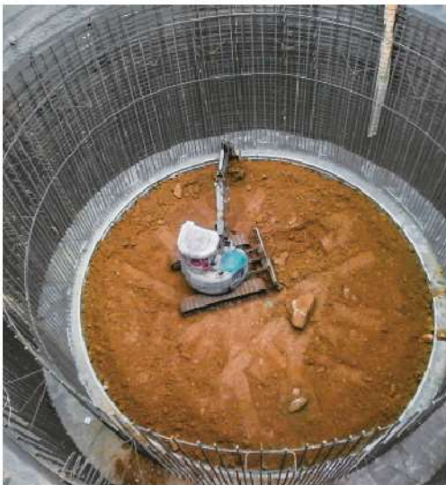
照0-40 井基中空土石方回填
