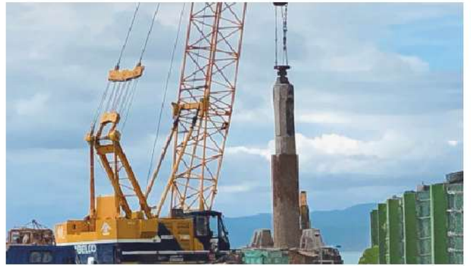
照2-43 棧橋基樁施作
