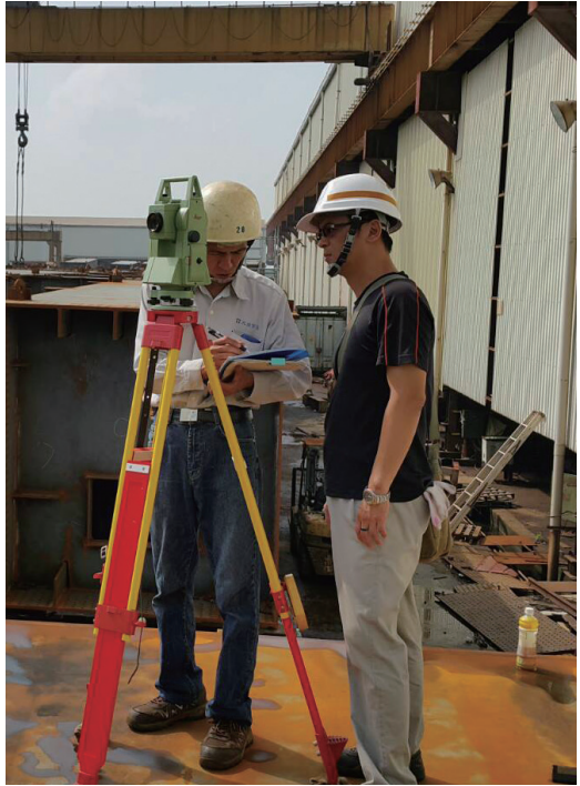
鋼構件假安裝查驗
