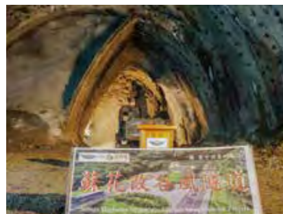
NN5海側導坑貫通
