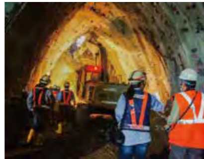
NN5海側導坑貫通
