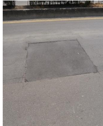
Fig. 2 Patching (taken by DGH)
