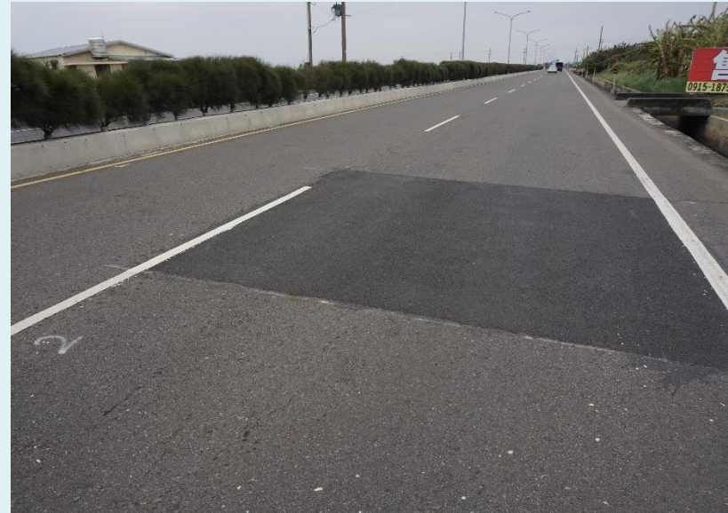
Severe pothole and good patching (Photo taken by DGH)
