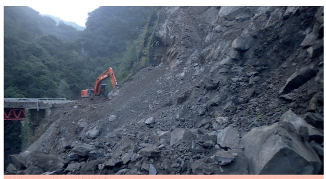
台7線32K+500處上邊坡災害搶修作業。 Emergency repair work on the slope of 32K + 500 section of the Provincial Highway No.7.
