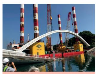
南方澳跨港大橋鋼拱吊離。 Nanfang 'ao Cross-harbour Bridge steel arch lift off.
