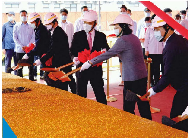
蔡英文總統主持祈福動土典禮。 President Tsai Ing-wen officiated at the groundbreaking and blessing ceremony.
