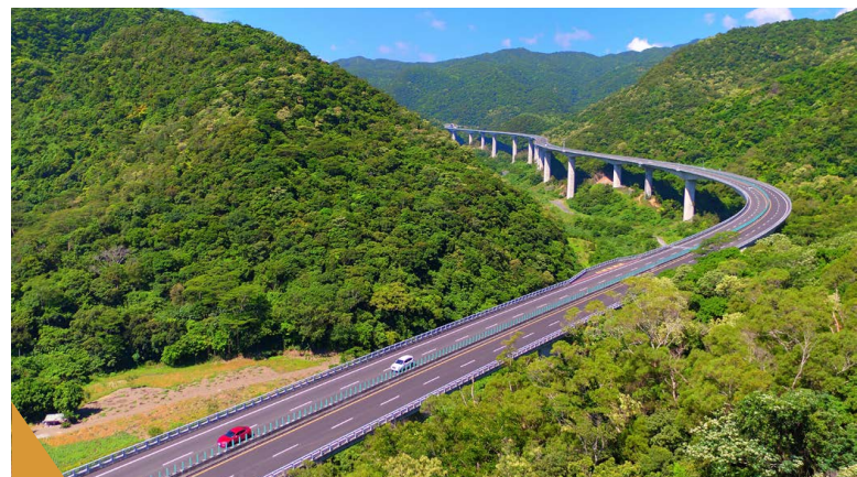
藏橋於林。 Hidden bridge in the forest.
