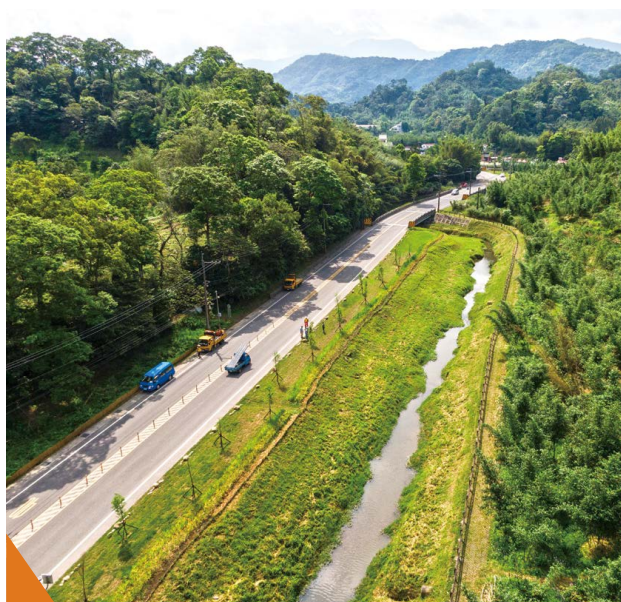
台7線8.8k水岸美景。 View of the 8.8k of Provincial Highway No.7.
