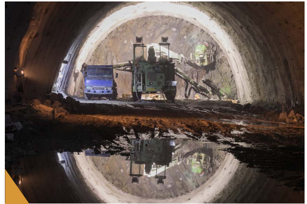
和中大清水段-施工之艱困。 Difficulty of construction Zhongda-Qingshui section.
