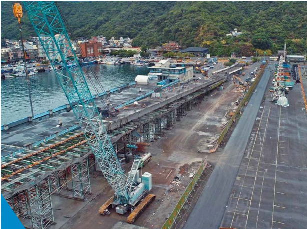
舊橋拆除。 Demolition of the old bridge.
