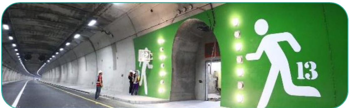
Figure 2-9 Picture Showing Emergency Pedestrian Cross-passage as Refuge in Tunnel
