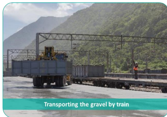
Figure 2-13 Utilization of Abandoned Railway Tunnel for Mucking by Rail Haulage
