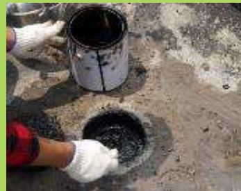
Coat the wall with emulsified asphalt and the soften the asphalt with a drying lamp.
