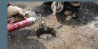
Drain the water in the pothole, and try the wall.
