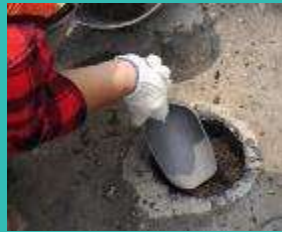
Chip the base flat before placing asphaltic sand
