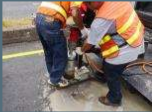
Core boring sampling.
